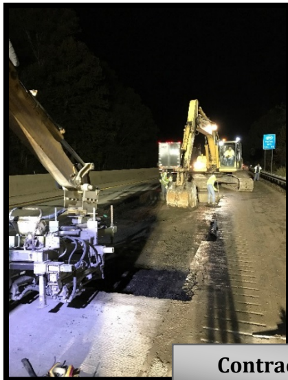
Contract 1A-18 Full Depth Concrete Repair
