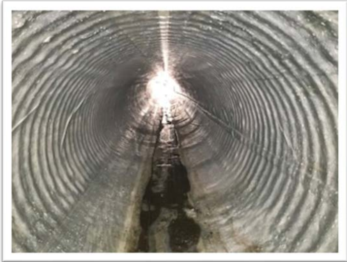
Culvert Liner Being Installed as a Method of Repair
