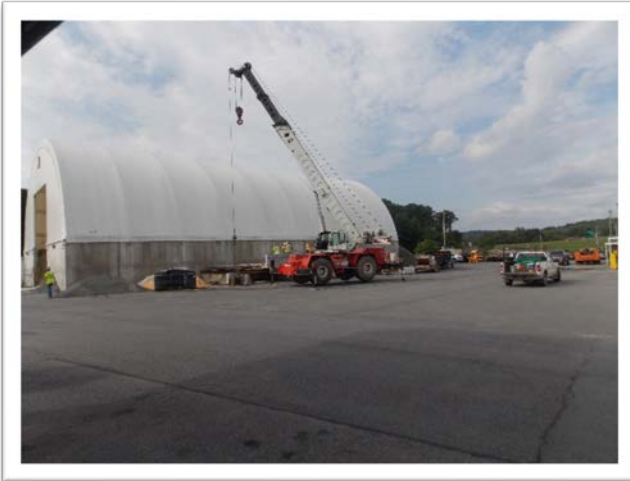
Pre-Cast Deck Panel Staging
