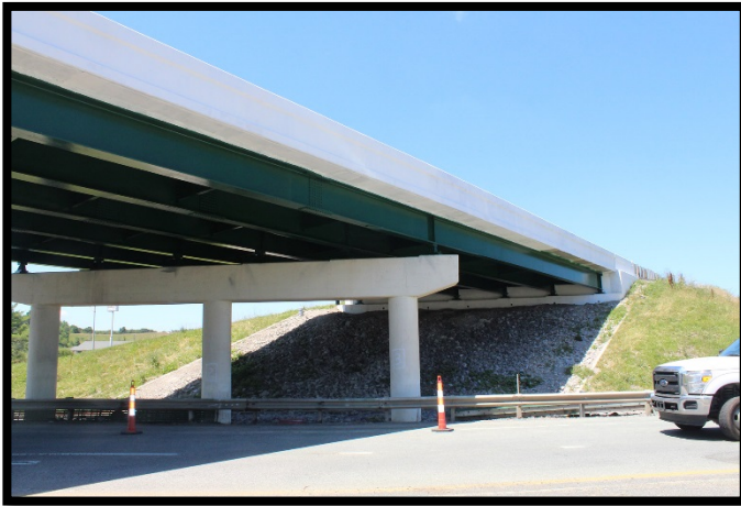
Bridge 3018S Full Repaint
