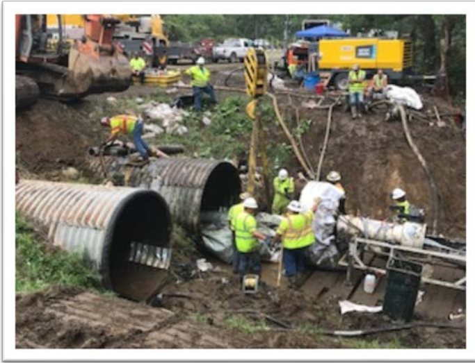
Culvert Liner Being Installed as a Method of Repair
