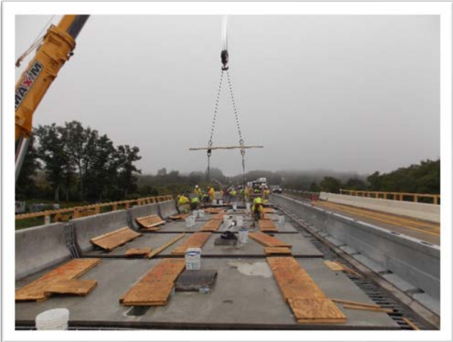
Pre-Cast Deck Panels in Place
