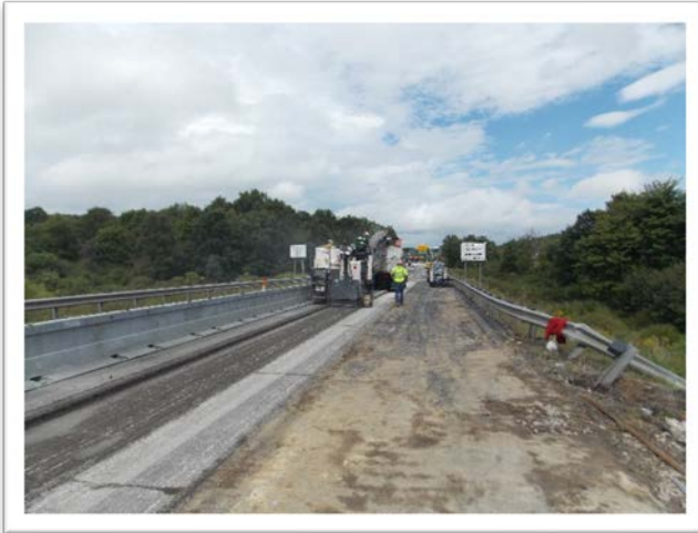
Milling of Approach Pavement
