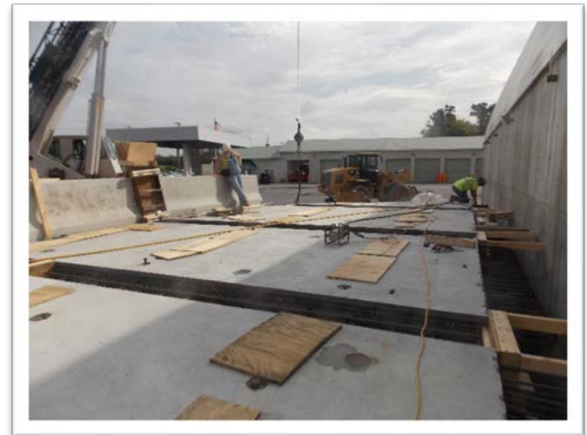
Off-Site Staging of the Pre-Cast Deck Panels
