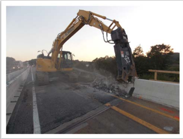
Demolition of the Existing Bridge
