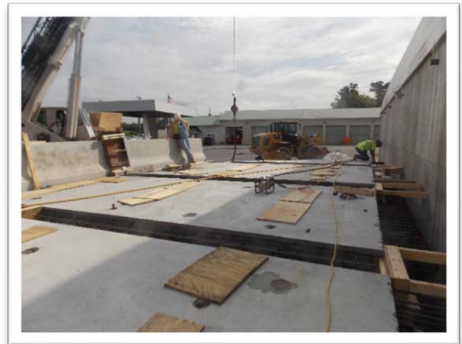
Off-Site Staging of the Pre-Cast Deck Panels
