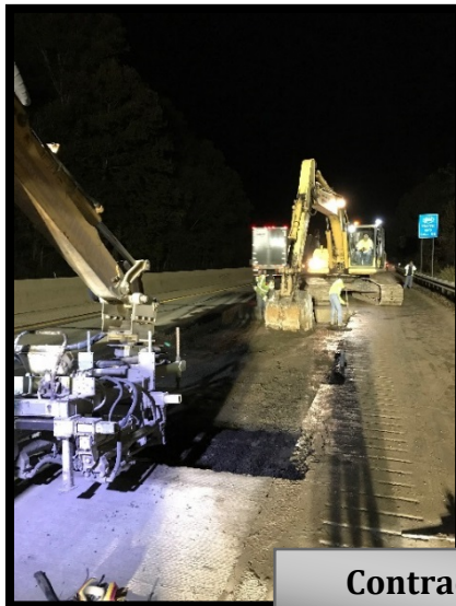
Contract 1A-18 Full Depth Concrete Repair
