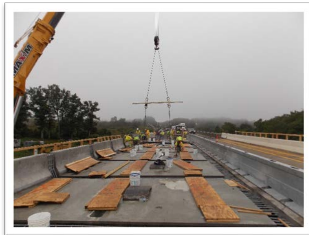
Pre-Cast Deck Panels in Place
