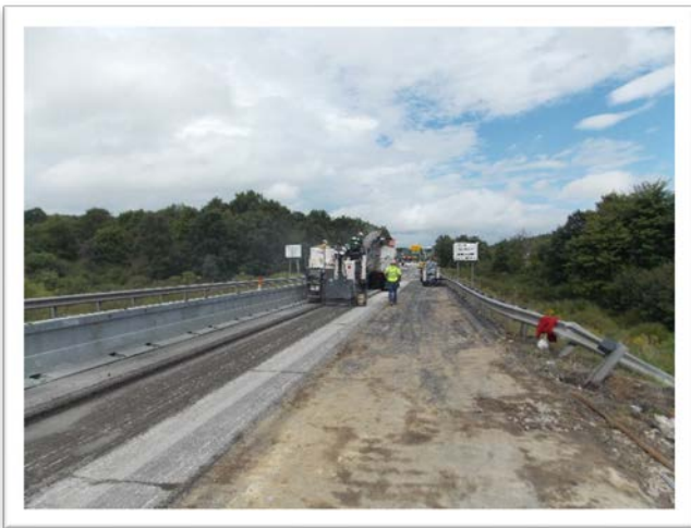
Milling of Approach Pavement
