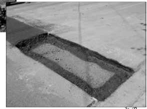
Patch Area After Tack
