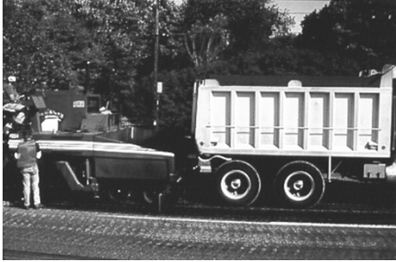
First contact with paver,... avoid bump!
