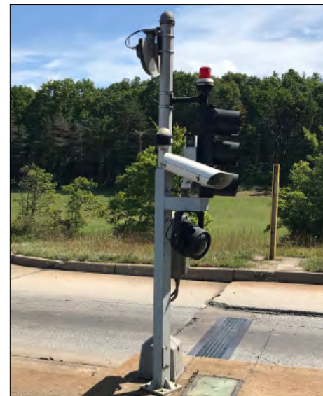
All lanes to include license plate image capture systems.
