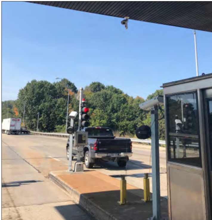
All lanes equipped with multi-protocol E-ZPass-compliant RFID AVI systems.
