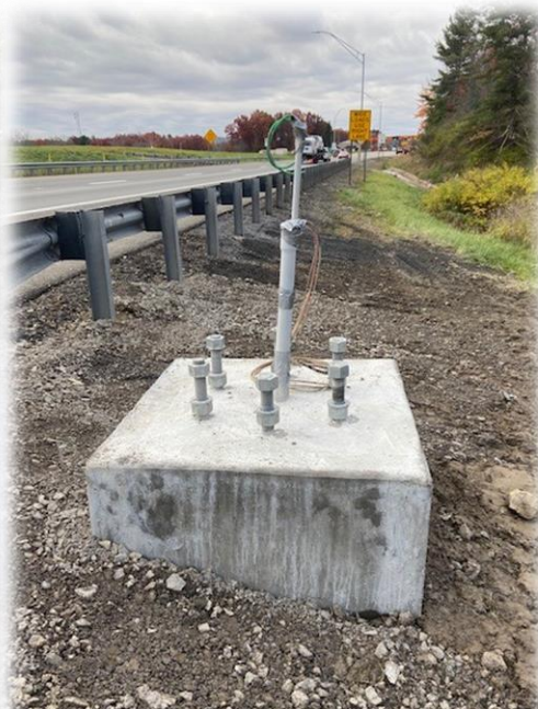
New Cantilever Sign Foundation Near Barrier A SB
