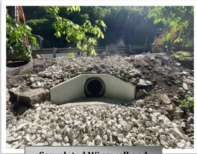
Completed Wingwall and Liner Installation
