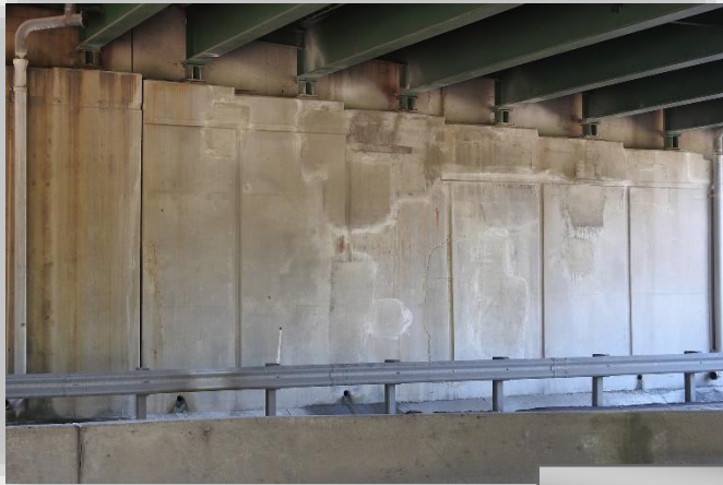
Abutment Repairs
