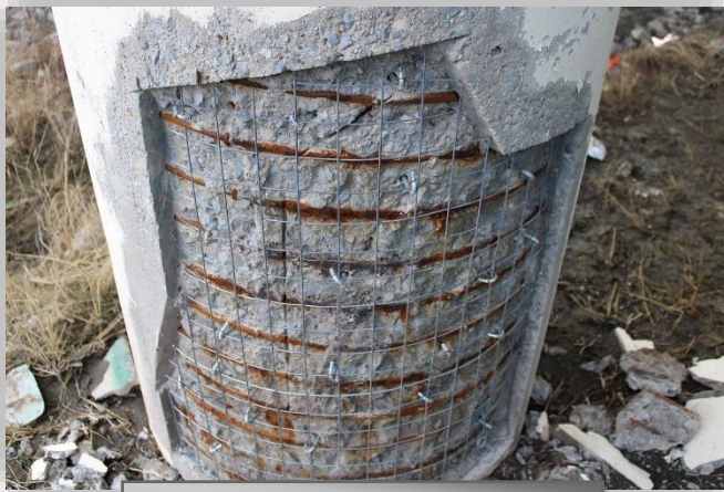
Pier Repairs Underway
