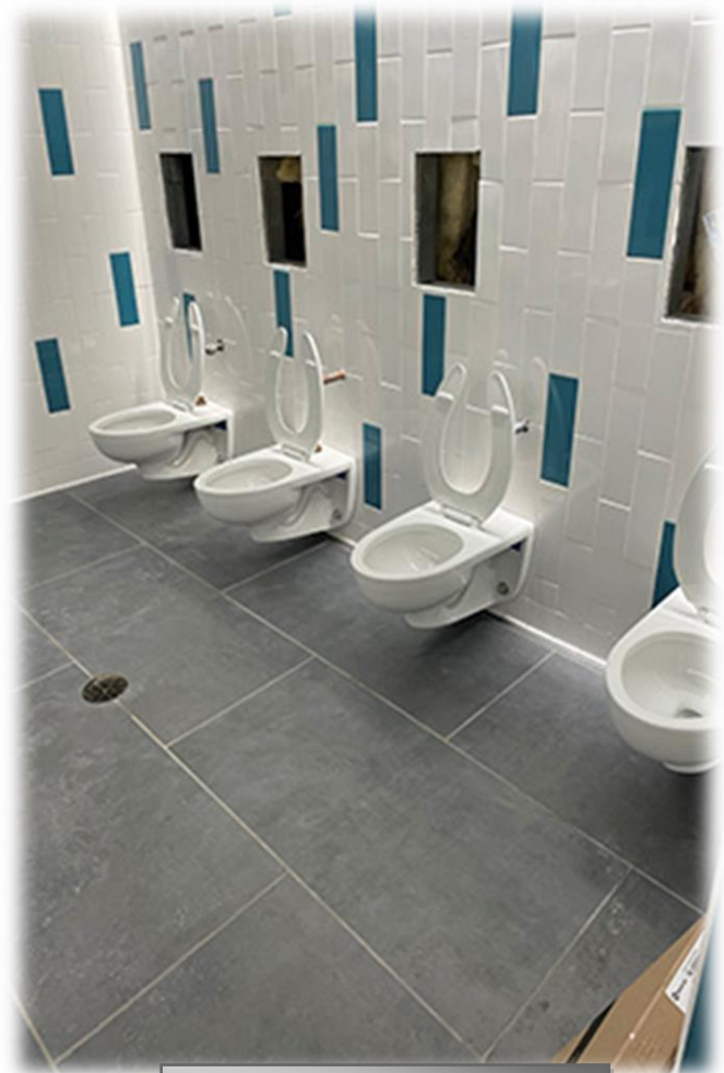
Floor and Wall Completed
