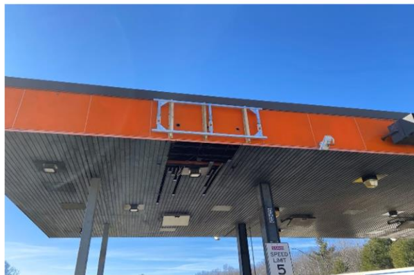
Toll Plaza Retrofit-Preparation for New VMS Boards
