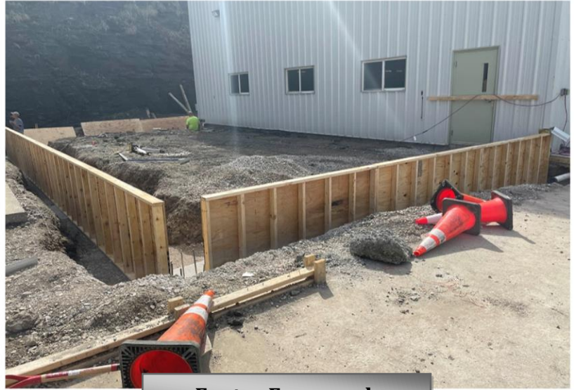
Footer Formwork
