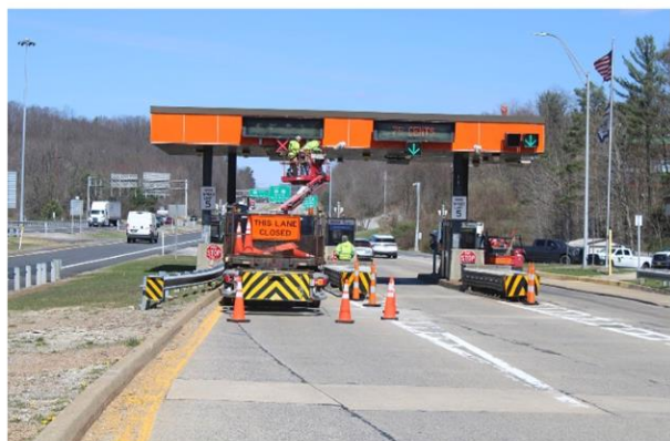
Toll Plaza Retrofit-Preparation for New VMS Boards
