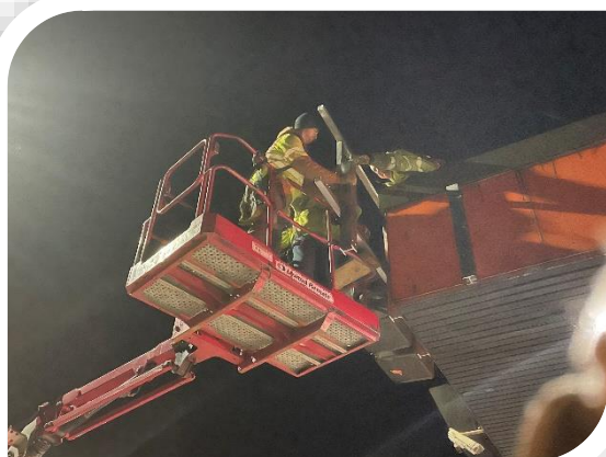
Toll Plaza Retrofit-Additional Canopy Support Columns Added
