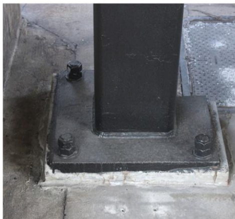
Toll Plaza Retrofit-Additional Canopy Support Columns Added
