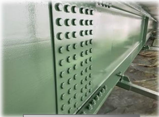
Bridge 3038 Paint Application
