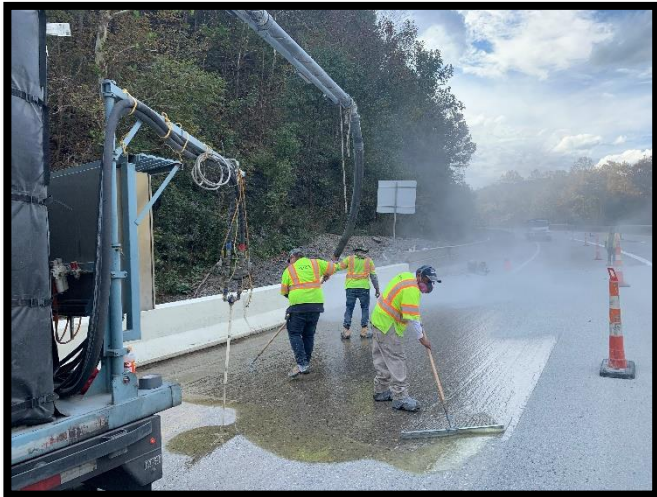
Bridge 3067S Protective Skid Resistant Deck Overlay
