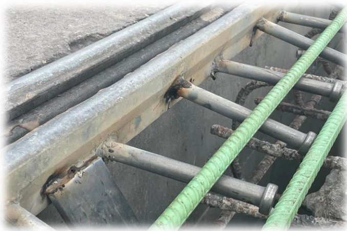
Typical Bridge Deck Joint Rehab/Replacement
