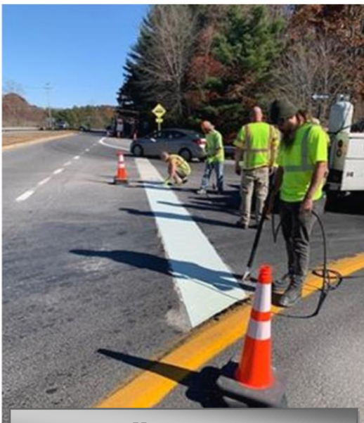
Installing Stop Bar
