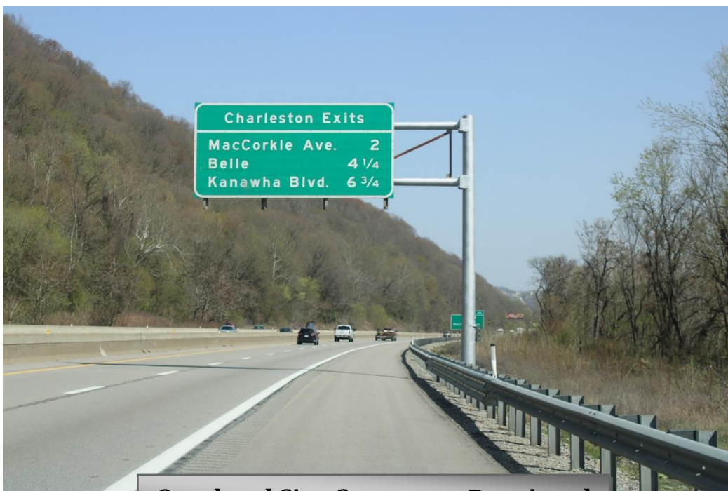
Overhead Sign Structures Repainted
