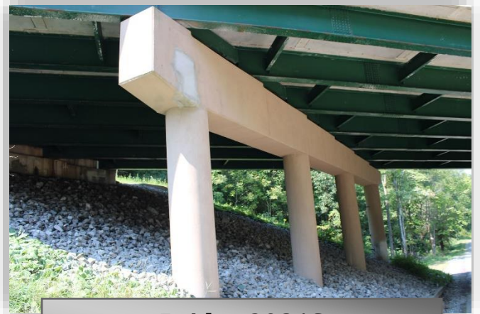
Bridge 3021S Pier Repairs Completed
