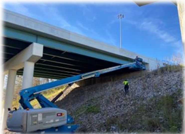
Coating Parapet Wall
