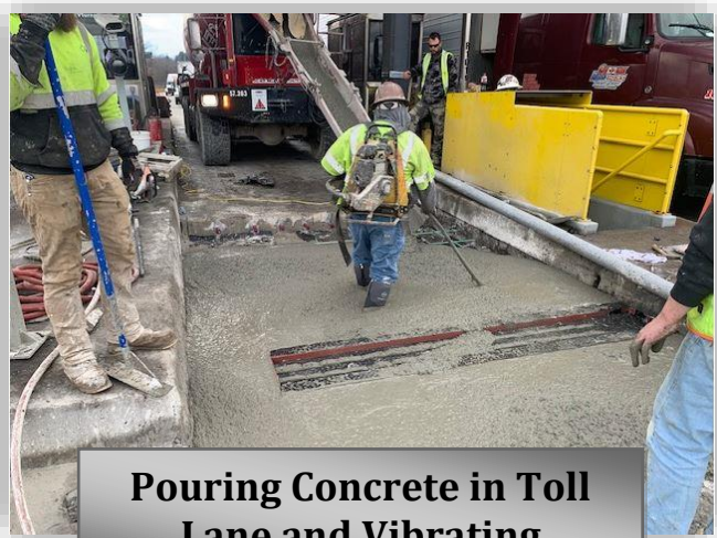
Finishing Concrete in Toll Lanes
