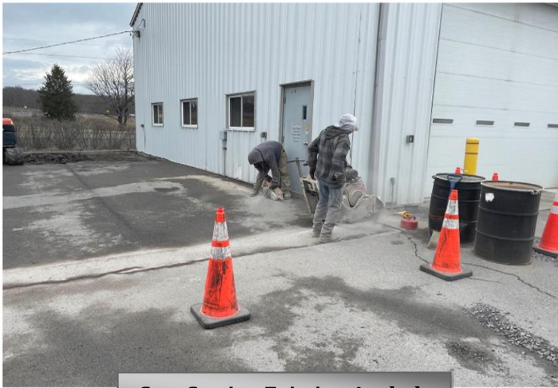
Saw Cutting Existing Asphalt
