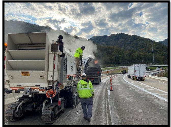
Bridge 3067S Protective Skid Resistant Deck Overlay
