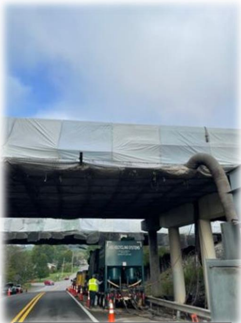
Bridge 3038 Containment Blasting
