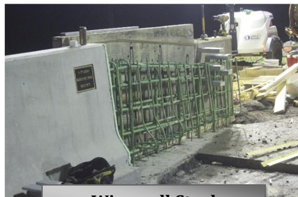
Wingwall Steel Reinforcement
