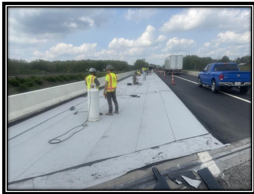
Applying Waterproofing
