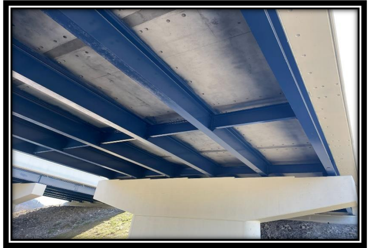
Steel and Concrete Coatings Applied
