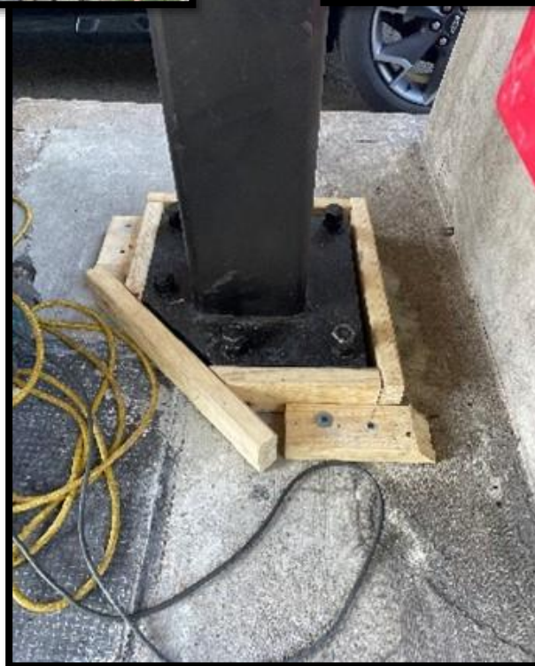
Setting Columns to Strengthen Toll Plaza Canopies
