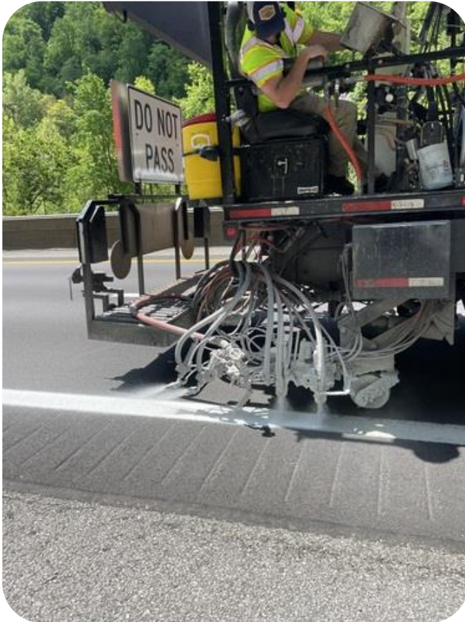
Installing Roadway Pavement Striping
