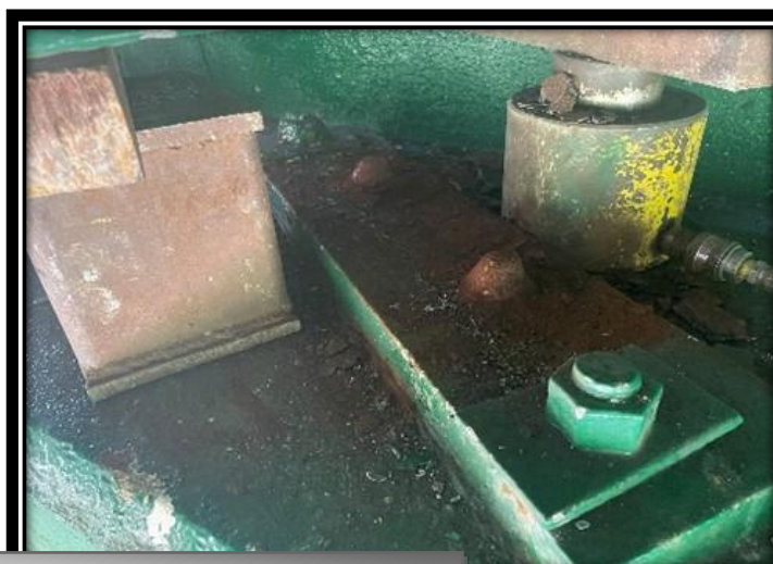
Bridge 3012S Resetting Bearings Abut 1
