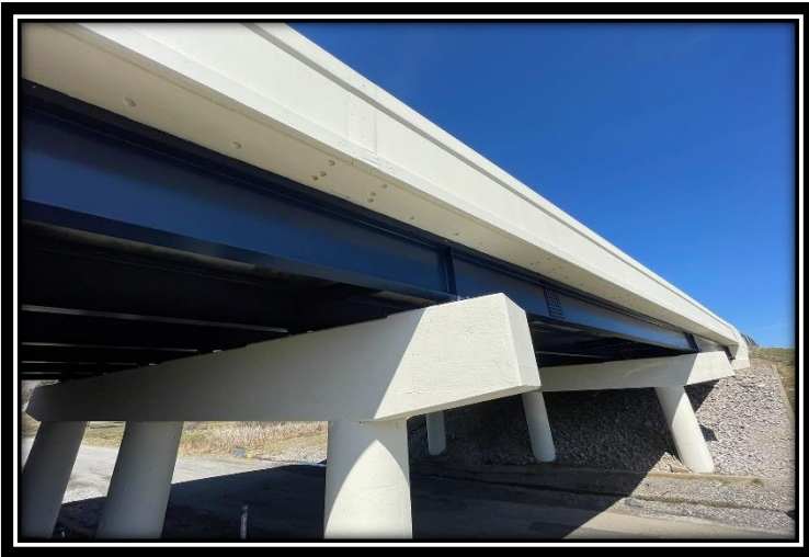
Steel and Concrete Coatings Applied
