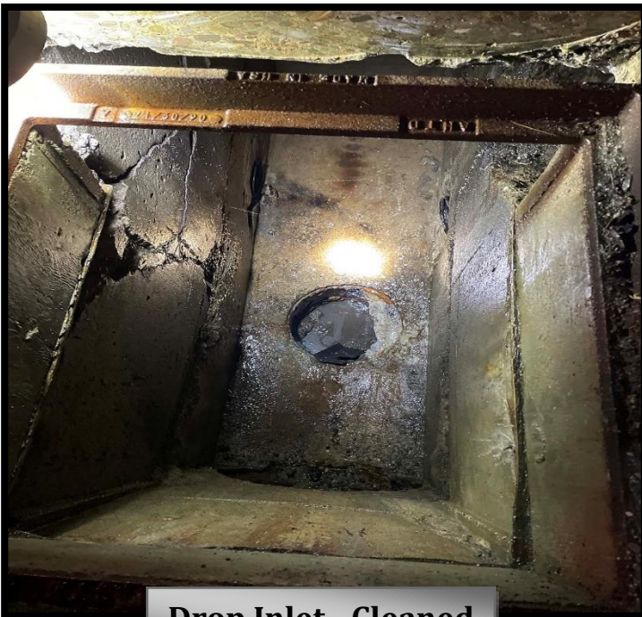
Drop Inlet - Cleaned
