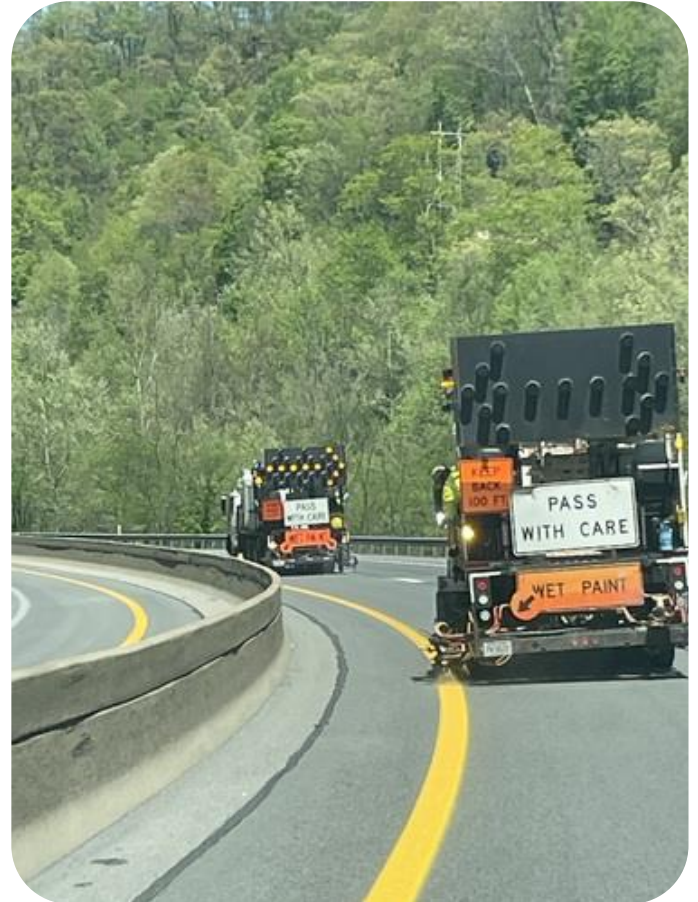
Installing Roadway Pavement Striping
