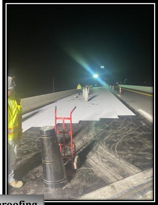
Applying Waterproofing
