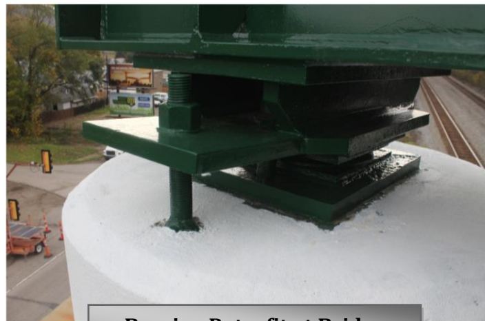
Bearing Retrofit at Bridge 3082N
