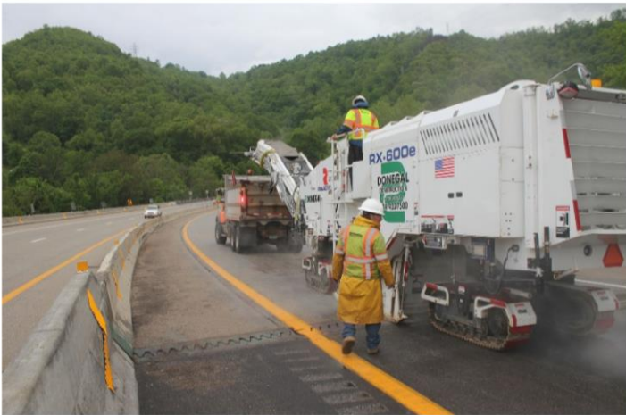
Deck Milling Prior to Resurfacing
