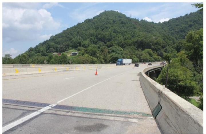
Bridge Deck Overlay with Non-Skid Surface
