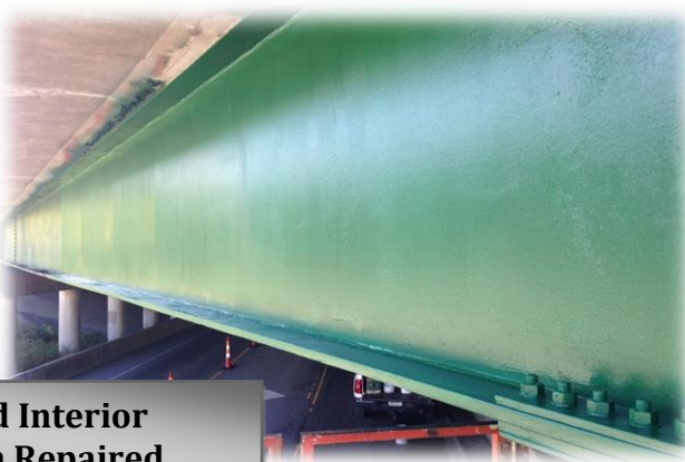
Repairing Fascia by Heat Straightening
