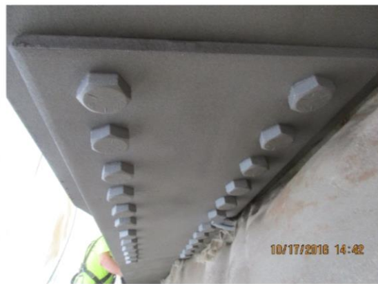
SP-10 Near White Metal Blast
