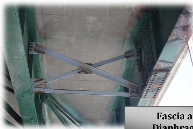
Repairing Fascia by Heat Straightening
