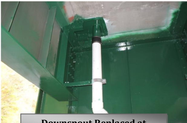
Downspout Replaced at Bridges 3082N/S
