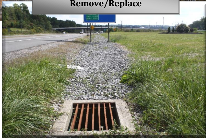
Culvert Repaired by Remove/Replace
