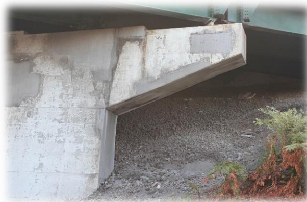
Delaminated Concrete Repaired on Pier
