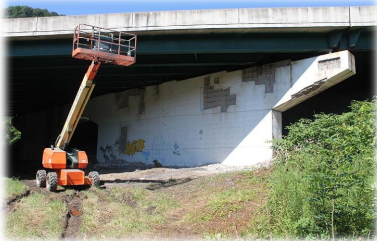
Pier Shotcrete Repair
