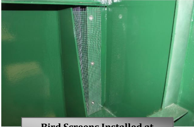
Bird Screens Installed at Bridges 3082N/S
