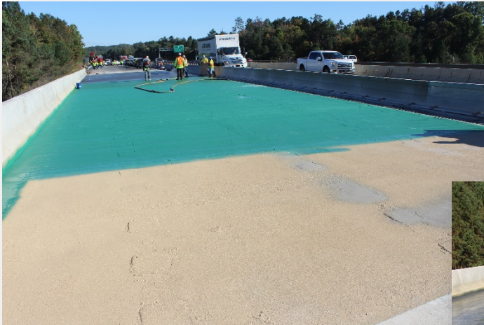
Waterproofing Membrane Application
