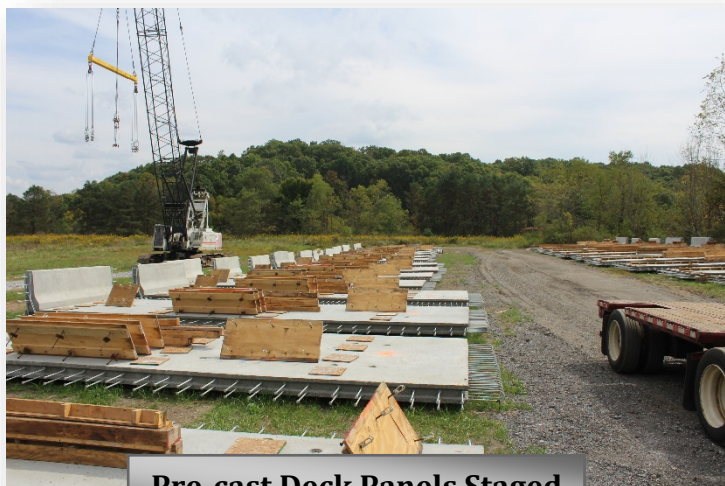
Pre-cast Deck Panels Staged
