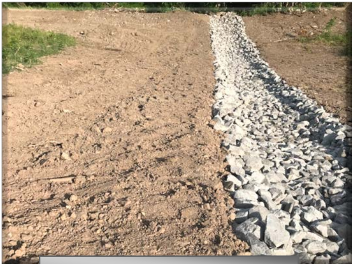
Dump Rock Gutter Installation
