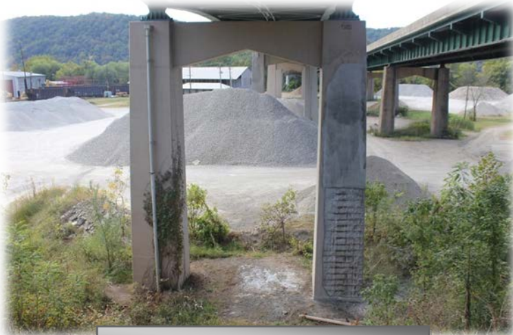
Pier Shotcrete Repair
