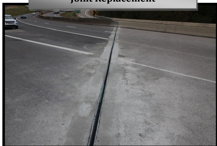
Bridge 3029 at Milepost 42.3 Joint Replacement
