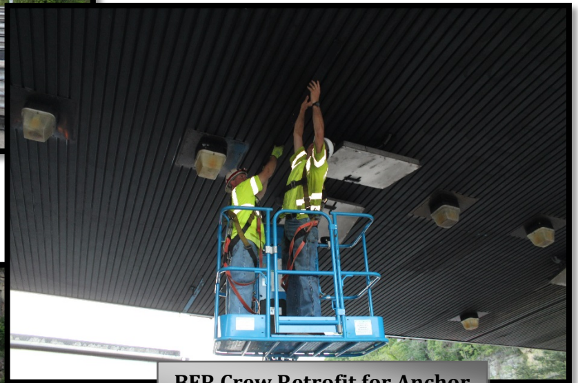
BFR Crew Retrofit for Anchor Bolt Installation
