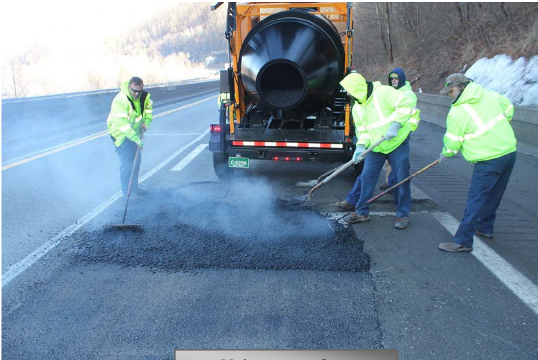
Maintenance Crew Patching Asphalt
