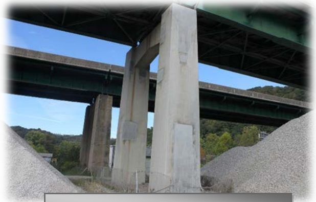
Delaminated Concrete Repaired on Pier
