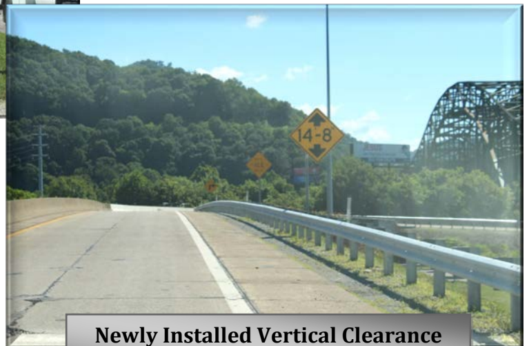
Newly Installed Vertical Clearance Signs at Bridge 3084 near Marmet
