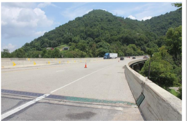
Bridge Deck Overlay with Non-Skid Surface
