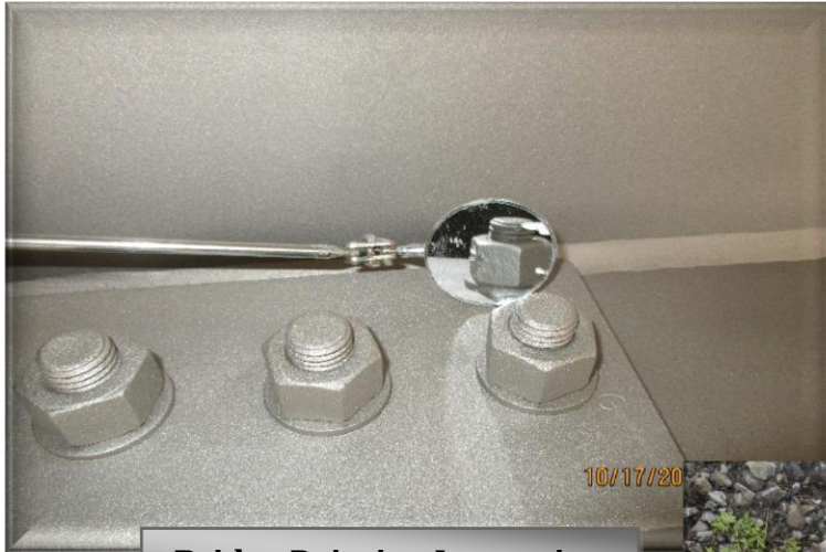
Bridge Painting Inspection
