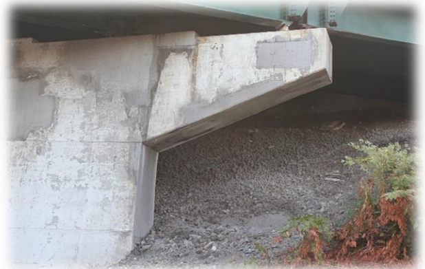
Delaminated Concrete Repaired on Pier
