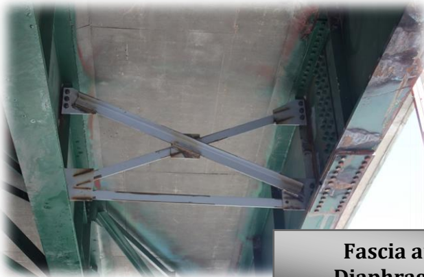
Repairing Fascia by Heat Straightening
