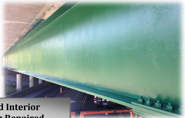
Repairing Fascia by Heat Straightening
