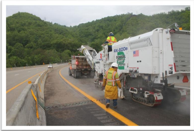
Deck Milling Prior to Resurfacing
