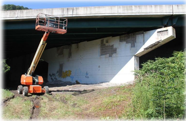
Pier Shotcrete Repair
