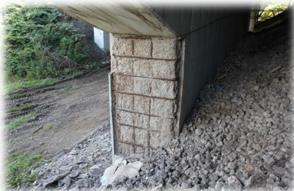
Delaminated Concrete Removed from Pier
