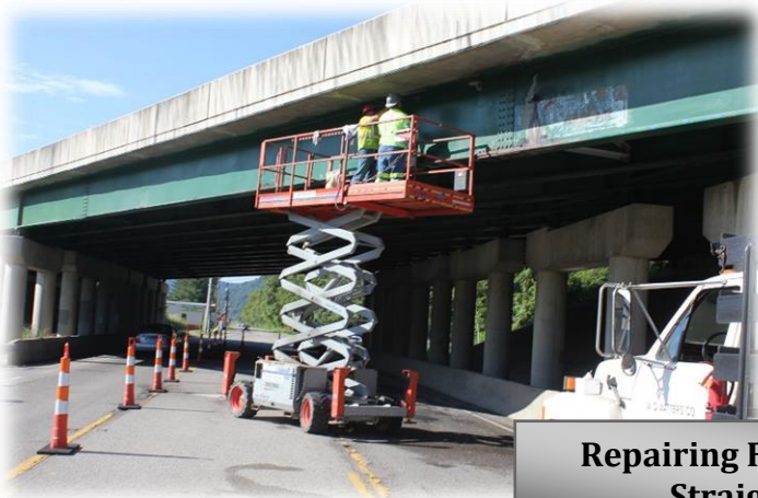
Distortion to Fascia from High Load Impact Damage
