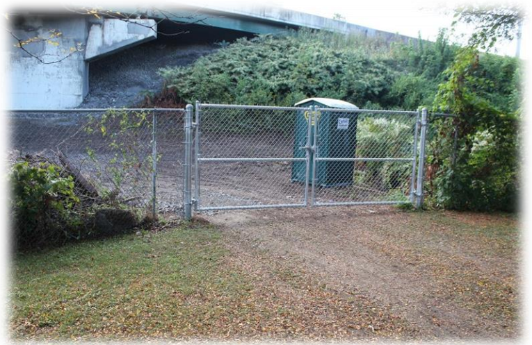
New Gate Installed by WVPA to Allow Access
