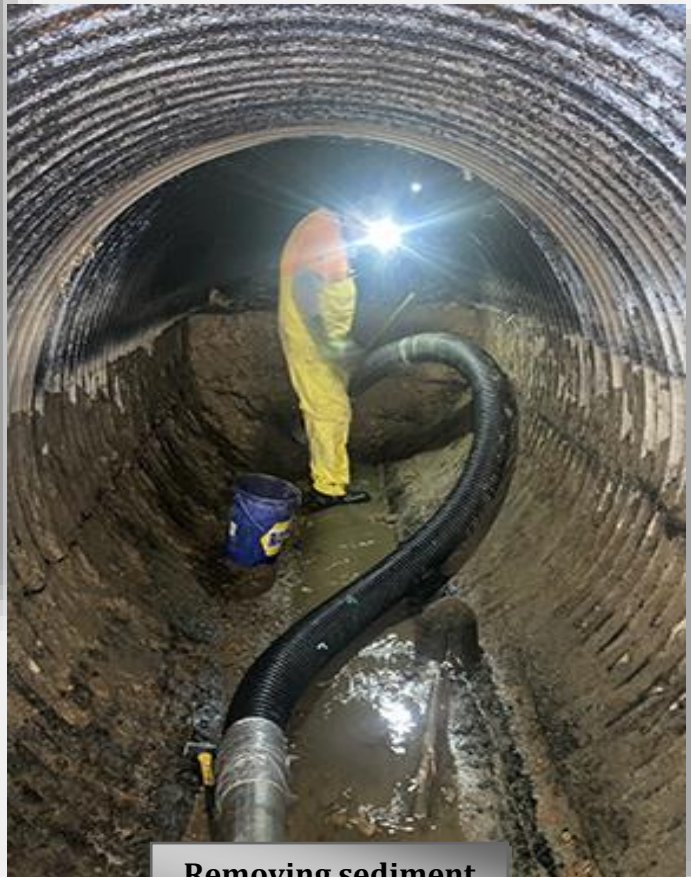
Removing sediment from culvert
