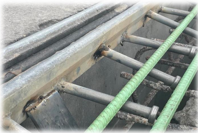
Typical Bridge Deck Joint Rehab/Replacement
