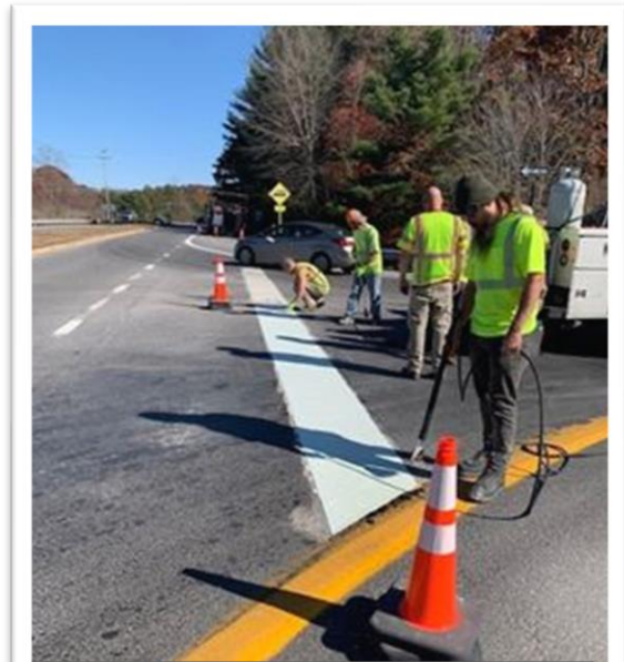
Installing Stop Bar
