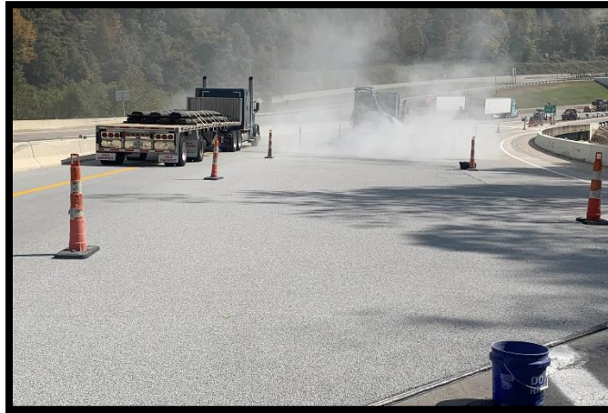
Bridge 3067S Protective Skid Resistant Deck Overlay
