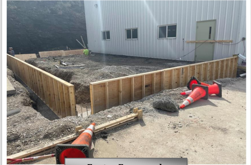
Footer Formwork
