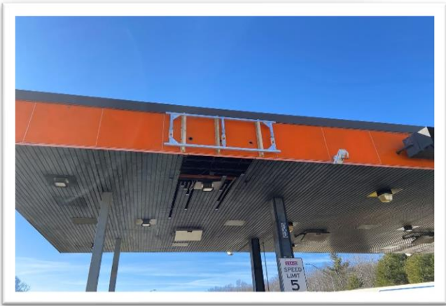
Toll Plaza Retrofit-Preparation for New VMS Boards
