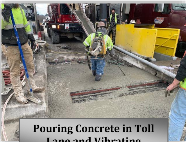
Finishing Concrete in Toll Lanes
