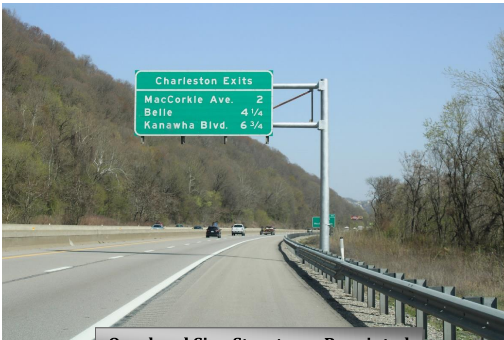
Overhead Sign Structures Repainted
