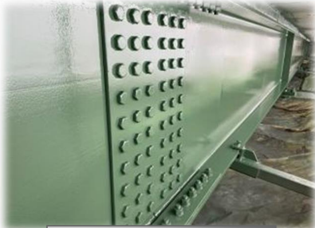
Bridge 3038 Paint Application
