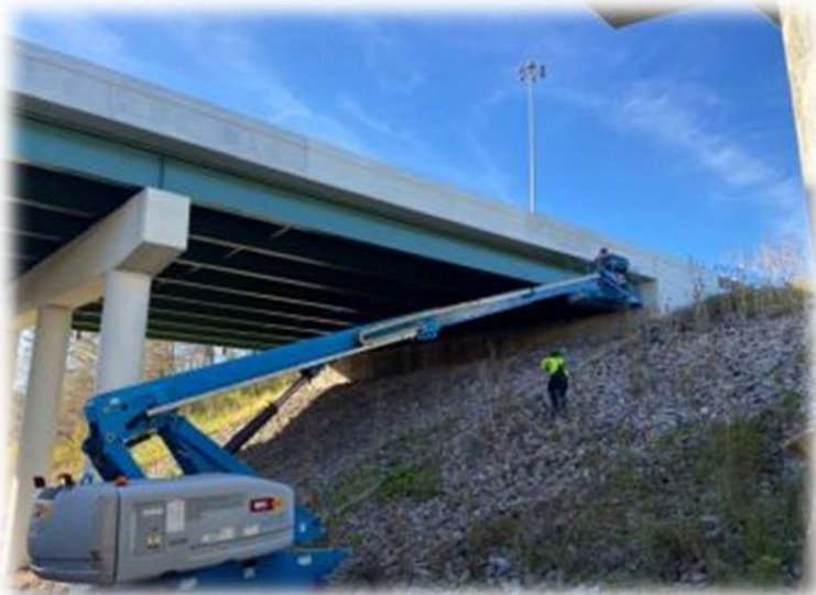
Coating Parapet Wall
