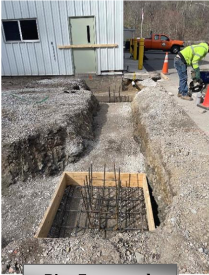
Pier Formwork
