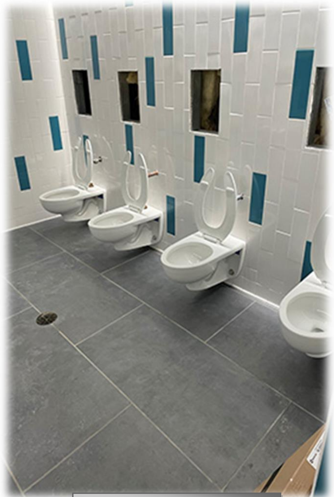
Floor and Wall Completed
