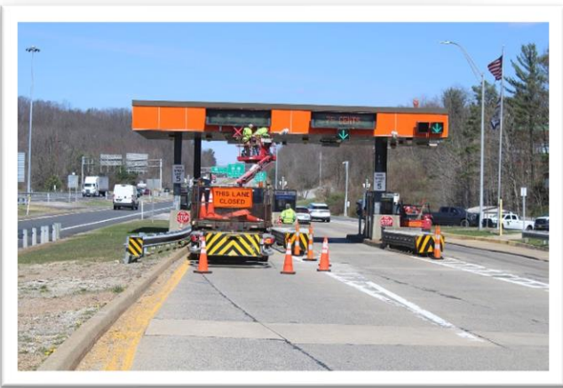
Toll Plaza Retrofit-Preparation for New VMS Boards
