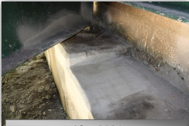
Bridge 3021N Abutment Repairs Completed
