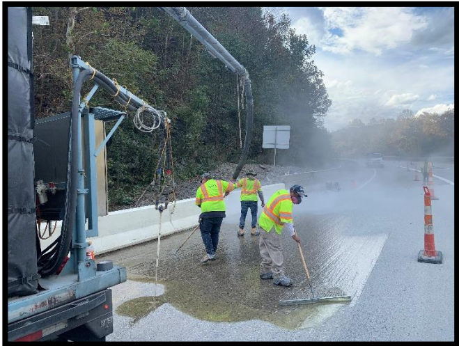
Bridge 3067S Protective Skid Resistant Deck Overlay
