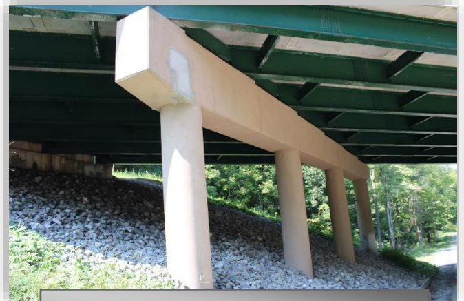
Bridge 3021S Pier Repairs Completed
