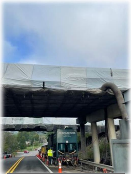
Bridge 3038 Containment Blasting
