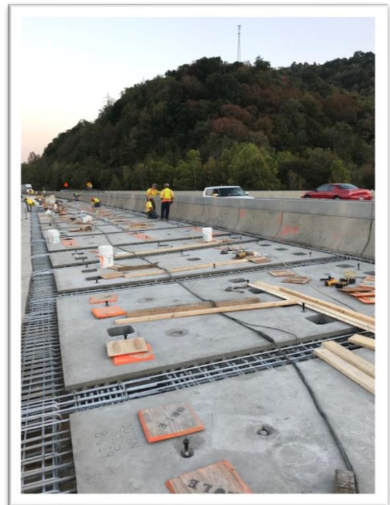
Pre-Cast Deck Panels in Place
