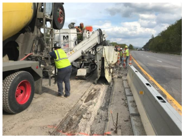
Slip Forming Median Wall
