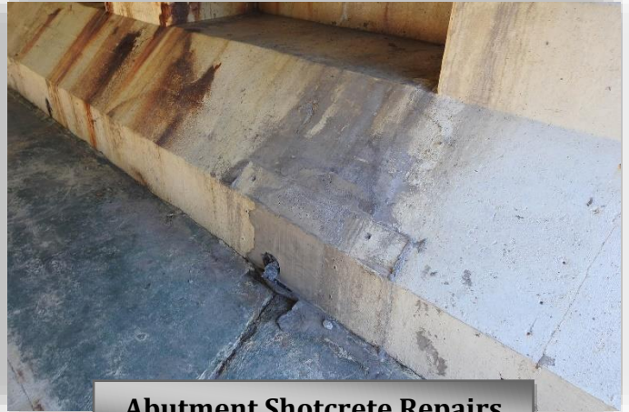
Abutment Shotcrete Repairs
