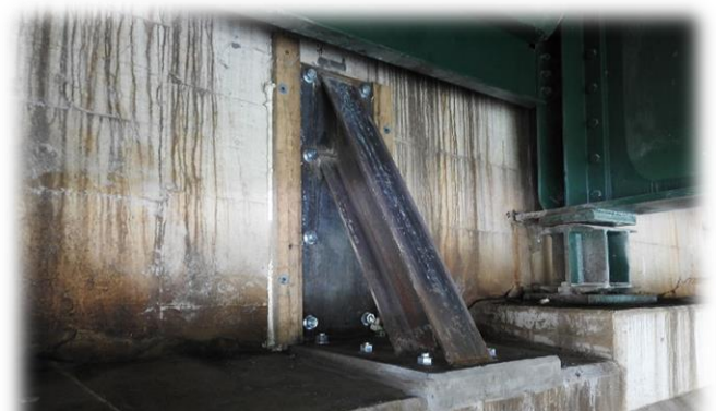
3076N S, Abutment Counterfort Retrofit
