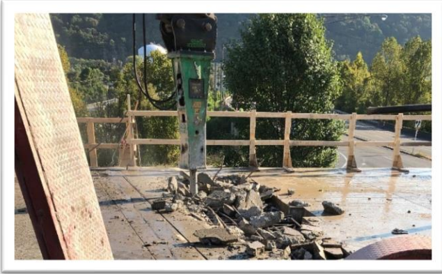
Demolition of the Existing Bridge
