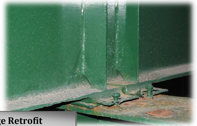
Bridge 3038N Bearing Retrofit
