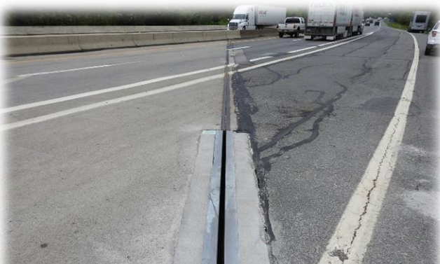
Bridge 3065S Deck Joint Replacement
