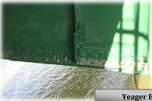
Bridge 3038N Bearing Retrofit
