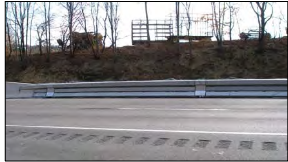
Typical Removable Concrete Median Barrier Gate
