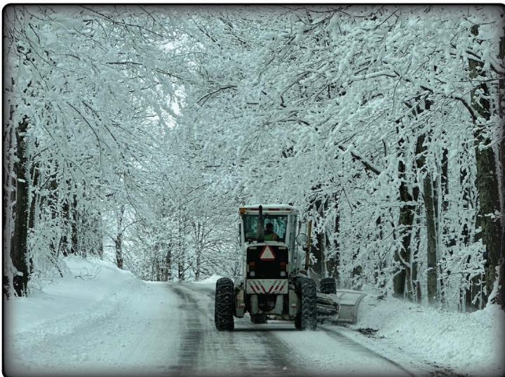
District 8, Jonathan Run Road, Tucker County.
