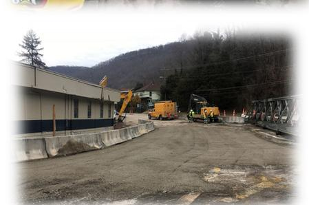
said crews were able to install a new, temporary drainage pipe inside the old structure. Beginning Tuesday, Jan. 3, 2023, crews began filling in the massive sinkhole with about 2,500 cubic yards of fill material. That's almost enough to fill an Olympic size swimming pool.
