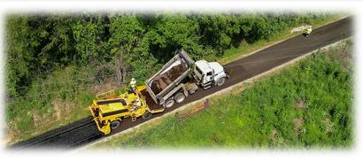
District 1 has a machine that can grind up the old asphalt into small particles, which can then be spread on the roadway like gravel.
