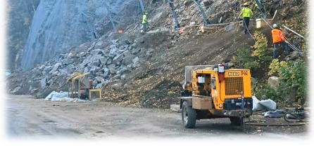
fences to catch any large rocks that may fall in the future. US 340 along the Shenandoah River built in was the mid-1950s. The cut slopes and exposed rock tower from 150 to more than 300 feet above the roadway.
