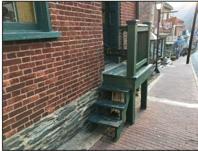
Figure 10: Wooden Steps on North Side of High Street
