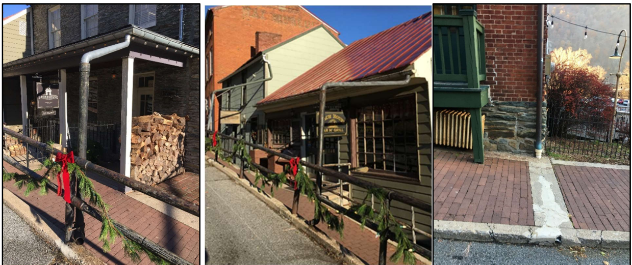
Figure 7: View of Downspouts on North Side of High Street
