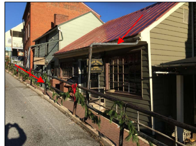
Figure 8 - Existing Roof Downspouts
