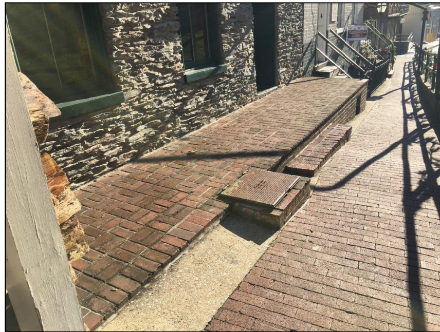
Figure 4 - Existing Sidewalk, East End
