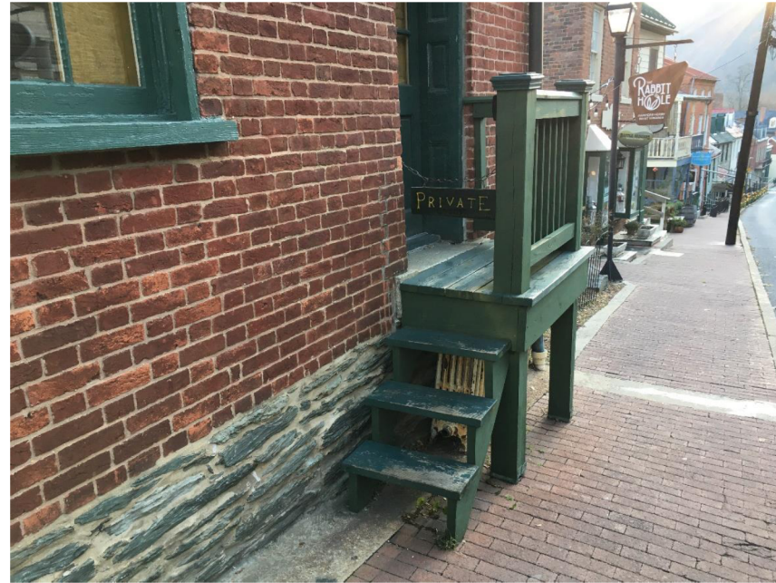
Figure 3 - Building Entrance, West (Upper End)
