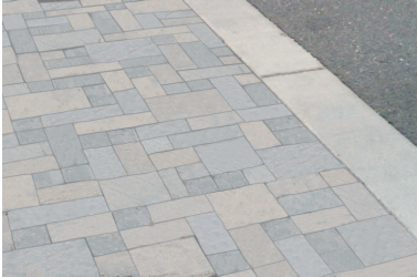
Crosswalk with Concrete Band and Venetian Stone Paver
