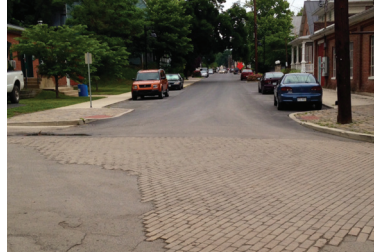
Fairfax Street & Wilkes Street
