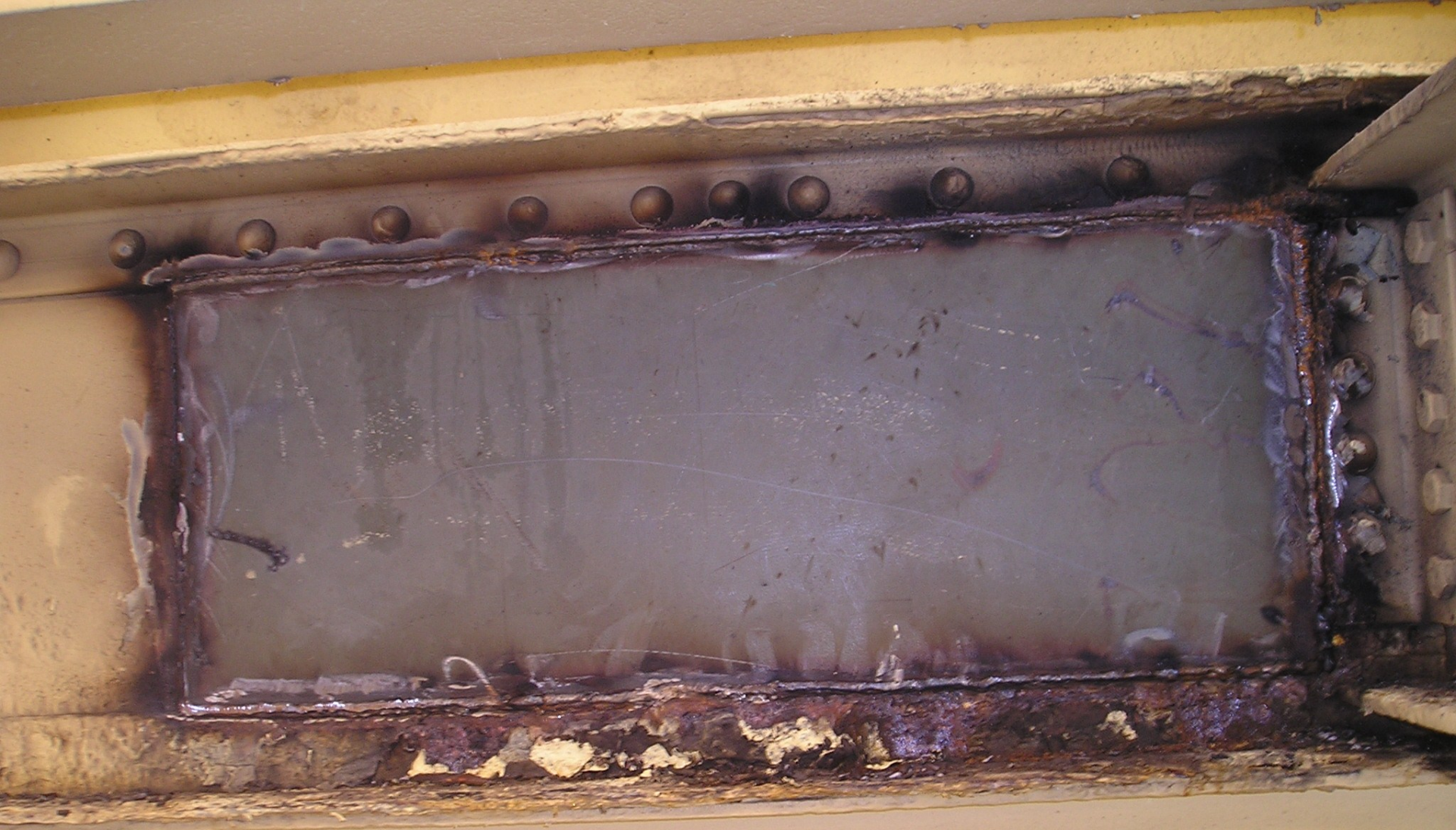
Additional floor beam repair as a result of the blasting
