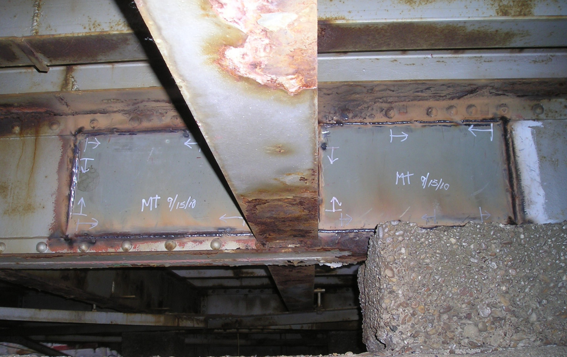
Patches to the floor beams
