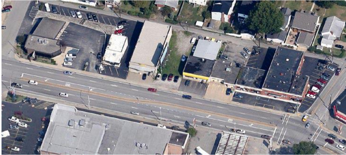
Existing excessive curb cuts
