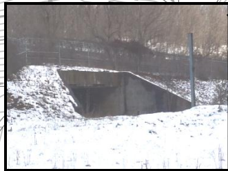
BOX CULVERT TUNNEL
