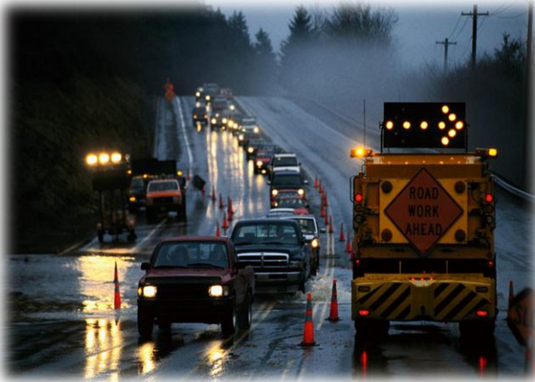
Work Zone Location/Status
