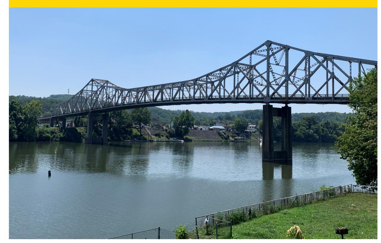
The existing bridge is a steel, riveted through truss bridge. It was previously determined eligible for listing in the National Register of Historic Places. Resources determined eligible or listed on the NRHP may also be protected by Section 4(f) of the U.S. Department of Transportation Act of 1966. Coordination with the State Historic Preservation Office (SHPO) has been, and will be, an important part of project planning in regard to potential adverse effects of alternatives being evaluated.
