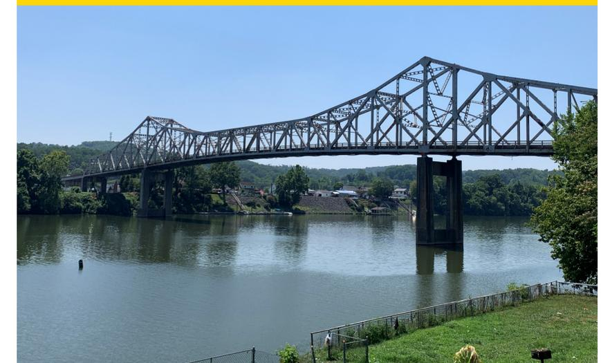
The existing bridge is a steel, riveted through truss bridge. It was previously determined eligible for listing in the National Register of Historic Places. Resources determined eligible or listed on the NRHP may also be protected by Section 4(f) of the U.S. Department of Transportation Act of 1966. Coordination with the State Historic Preservation Office (SHPO) has been, and will be, an important part of project planning in regard to potential adverse effects of alternatives being evaluated.
