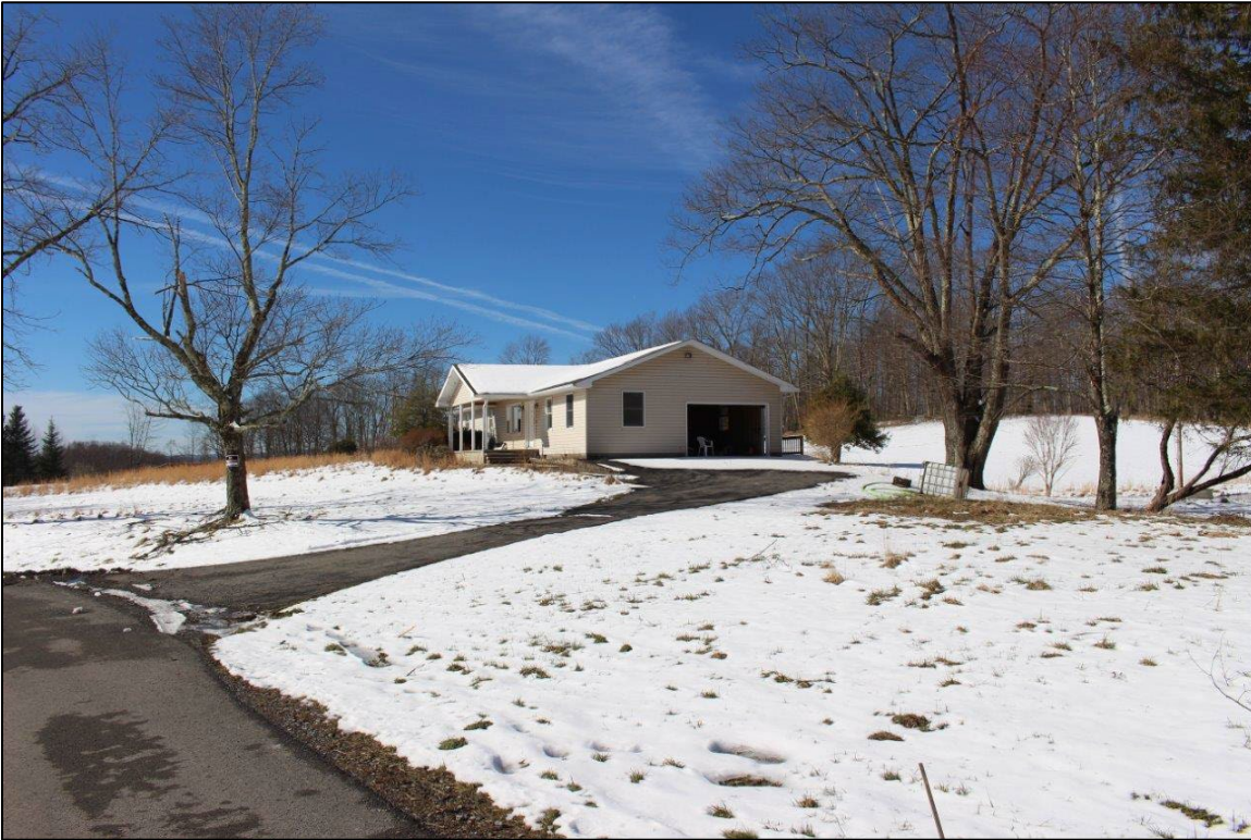
Photo 1. Gnegy/Spradlin/Graham House showing general view of property, facing southwest.
