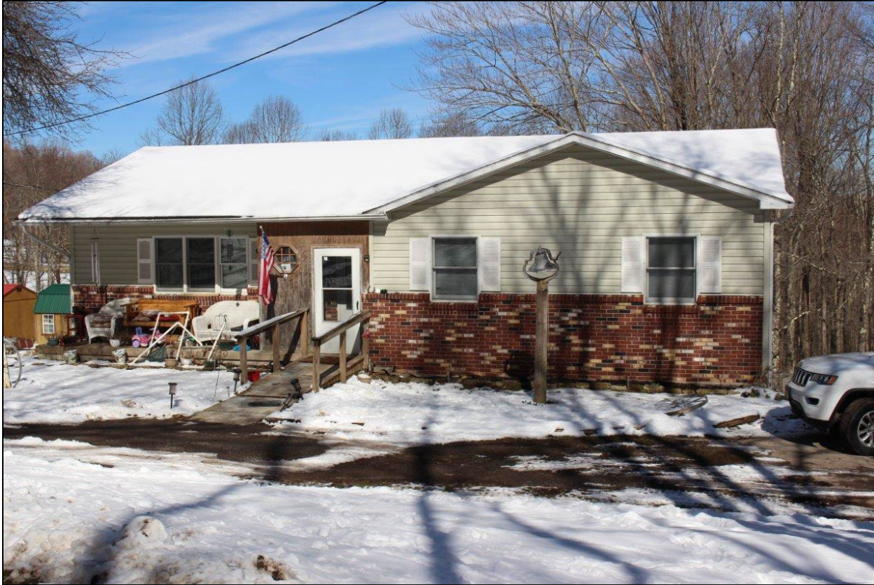
Photo 1. Sharp House showing south (front) façade of dwelling, facing north.
