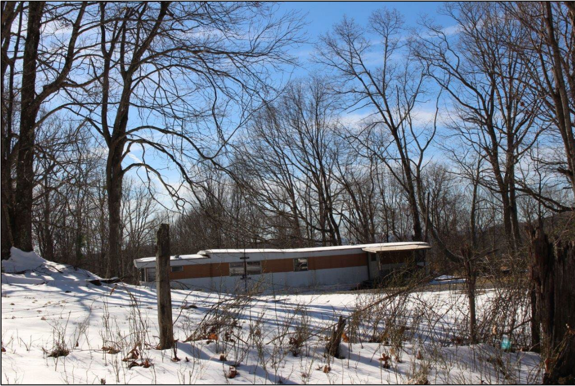
Photo 3. Minear Trailer showing northeast (front) façade, facing northwest.
