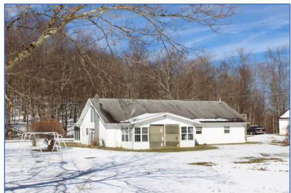
Photo 18. TU-1122, Snyder-Davis House.
