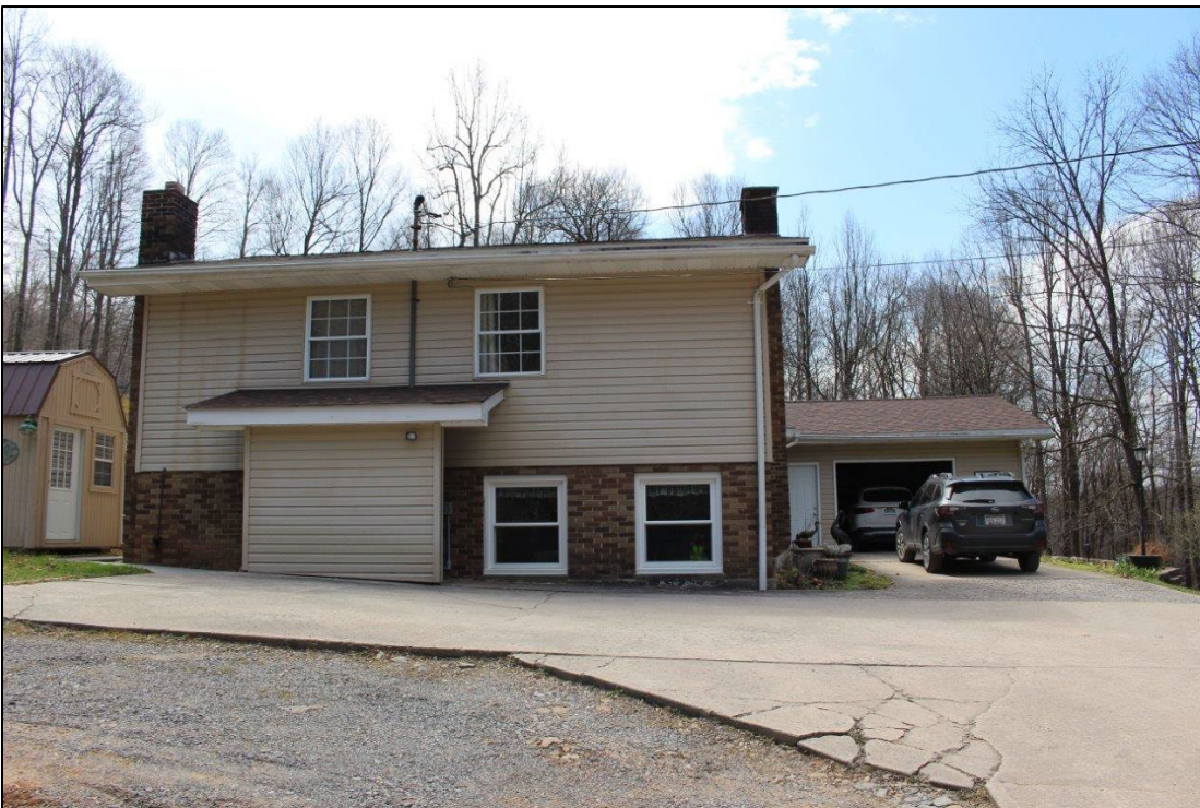
Photo 2. Ernest and Erma Snyder House showing northeast (front) façade, facing southwest.
