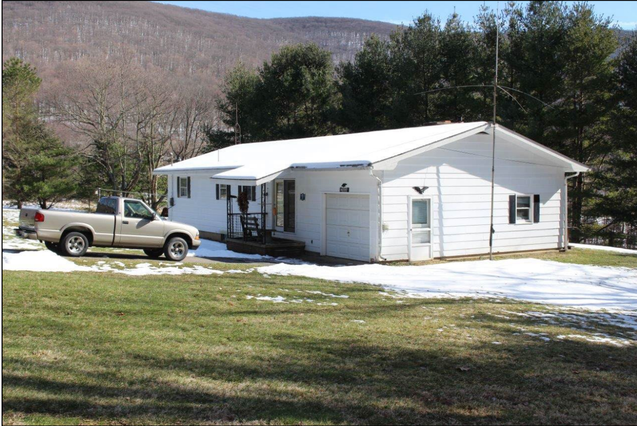
Photo 1. Phillip D. Oaster House showing northeast (rear) and northwest (side) façades, facing southeast.
