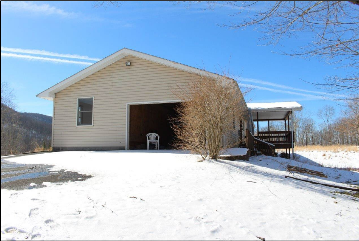
Photo 3. Gnegy/Spradlin/Graham House showing northeast (side) façade, facing southwest.
