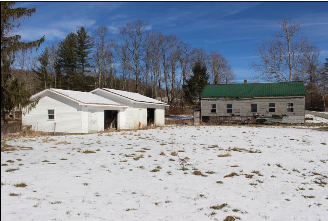
Photo 8. Gnegy/Spradlin/Graham House showing southwest (side) and southeast (front) façades of abandoned garage, and southwest (side) façade of abandoned dwelling (TU-0616), facing north.
