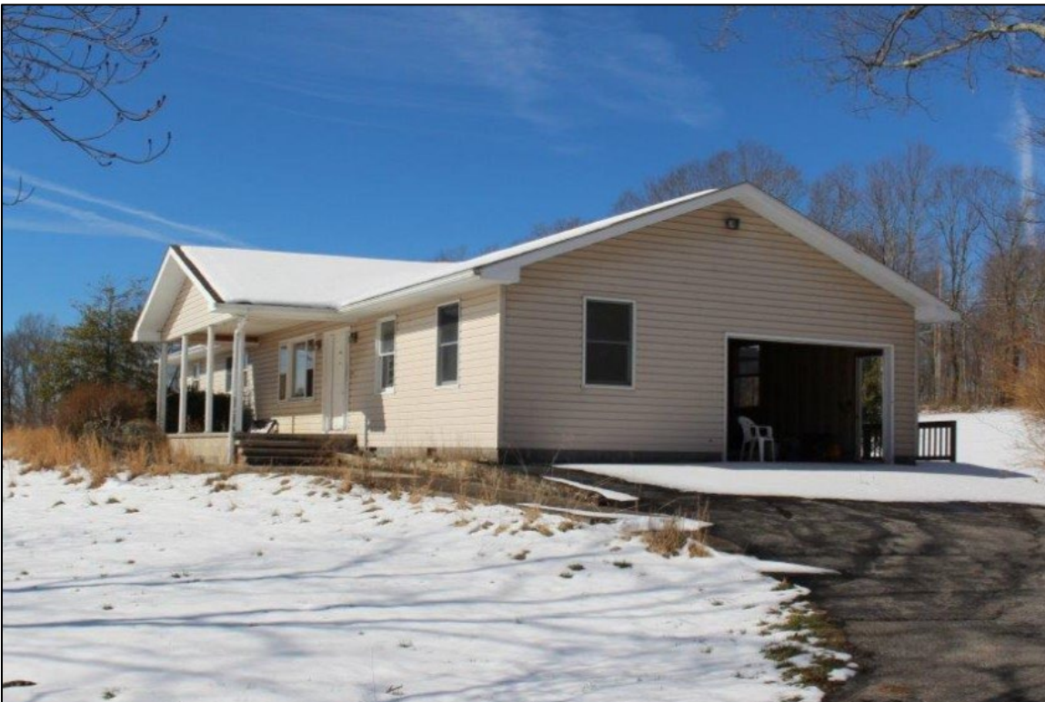
Photo 2. Gnegy/Spradlin/Graham House showing southeast (front) and northeast (side) façades, facing southwest.
