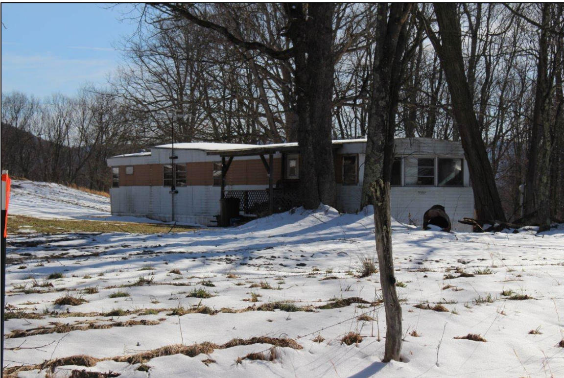
Photo 4. Minear Trailer showing northeast (front) and northwest (side) façades, facing southwest.
