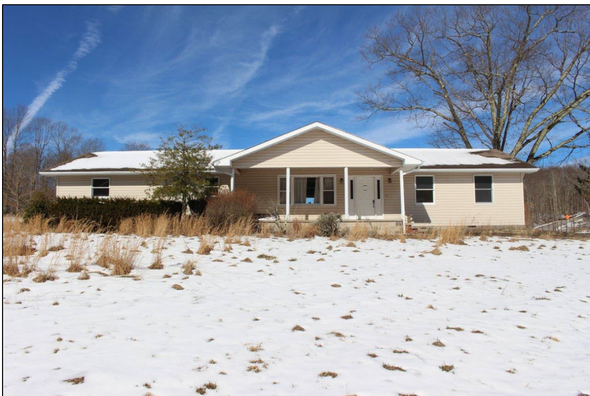
Photo 6. Gnegy/Spradlin/Graham House showing southeast (front) façade, facing northwest.
