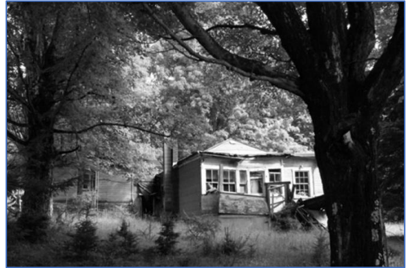
Photo 16. TU-0618, William Collette House – DEMOLISHED , 159 Silver Fox Road, 2015
