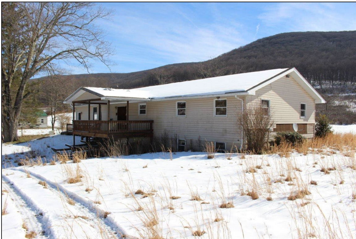
Photo 5. Gnegy/Spradlin/Graham House showing northwest (rear) and southwest (side) façades, facing east.
