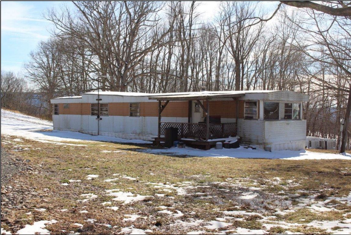
Photo 1. Minear Trailer showing northeast (front) and northwest (side) façades, facing southwest.
