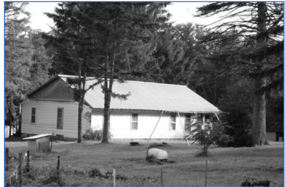
Photo 14. TU-617, Donald Gnegy House – DEMOLISHED, photo ca. 2015.
