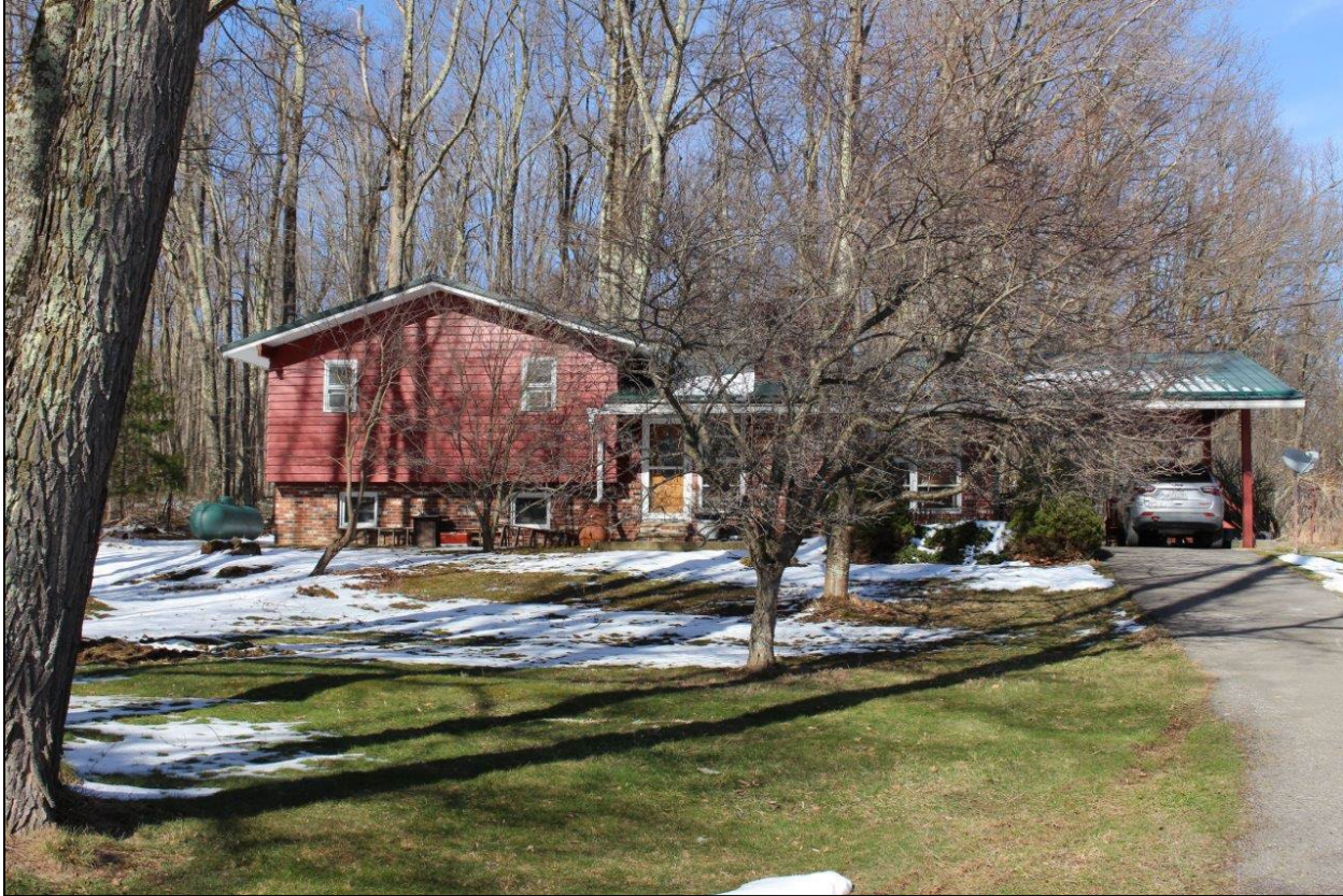
Photo 1. Gary Gwinn House showing southwest (front) façade, facing northeast.
