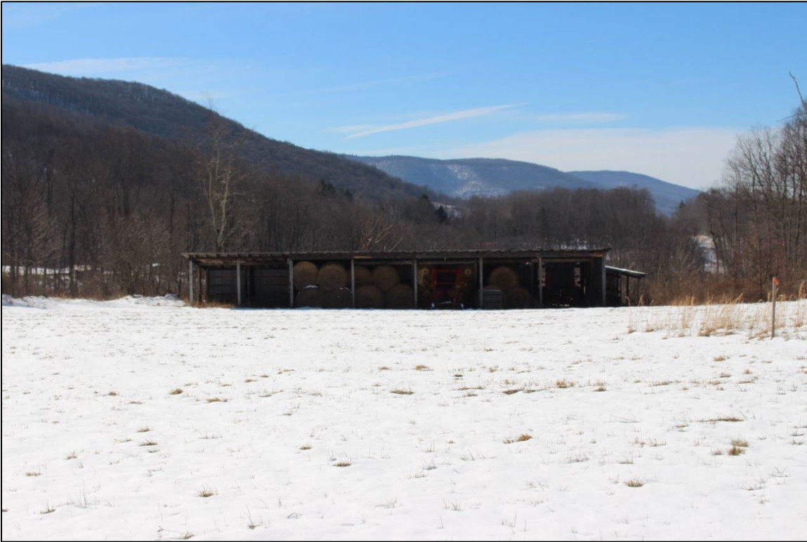
Photo 11. Gnegy/Spradlin/Graham House showing northeast (front) façade of tractor shed at southern end of property, facing south.
