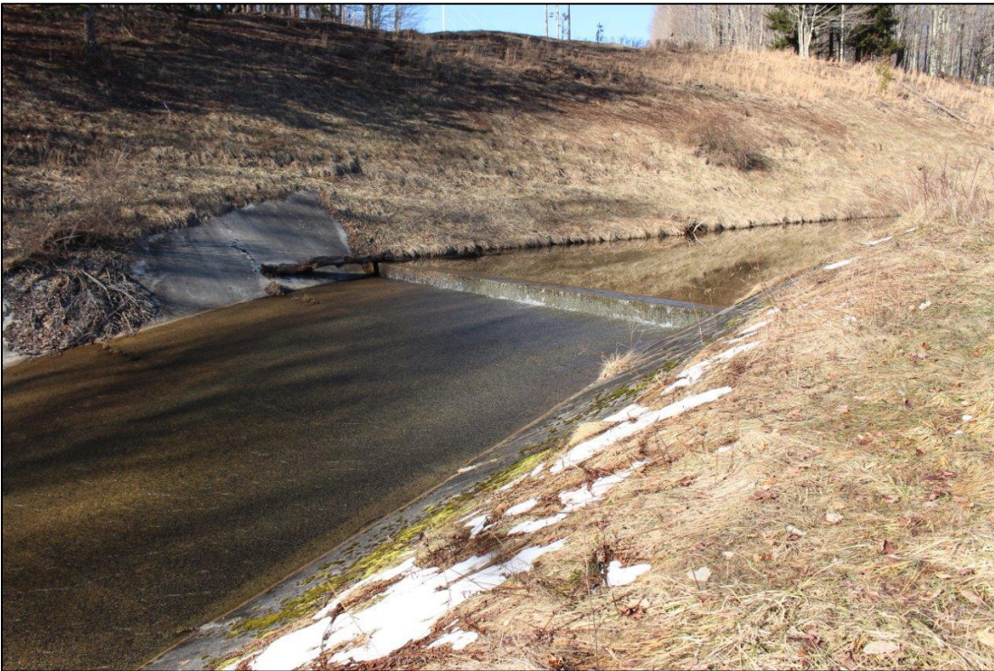
Photo 4. Thomas Reservoir Dam showing detail view of stepped concrete spillway, facing north.
