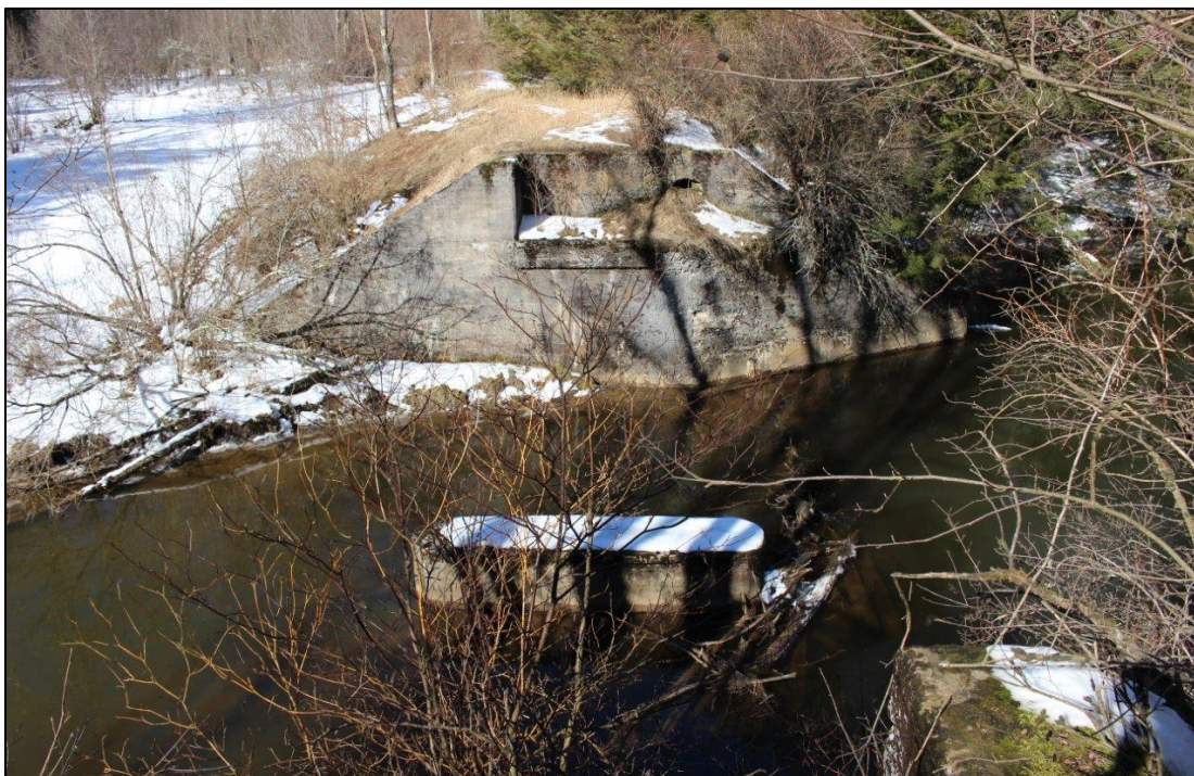
Photo 2 West Virginia & Central Pittsburg Railway, Pierce Branch showing concrete wingwall and pier remnant of former railroad bridge over the North Fork of the Blackwater River, facing northwest.
