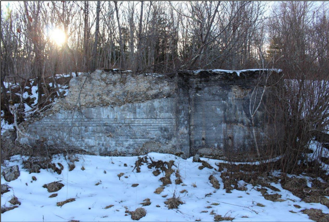
Photo 7. Building Ruins showing poured concrete wall remnant along west side of site, facing west.
