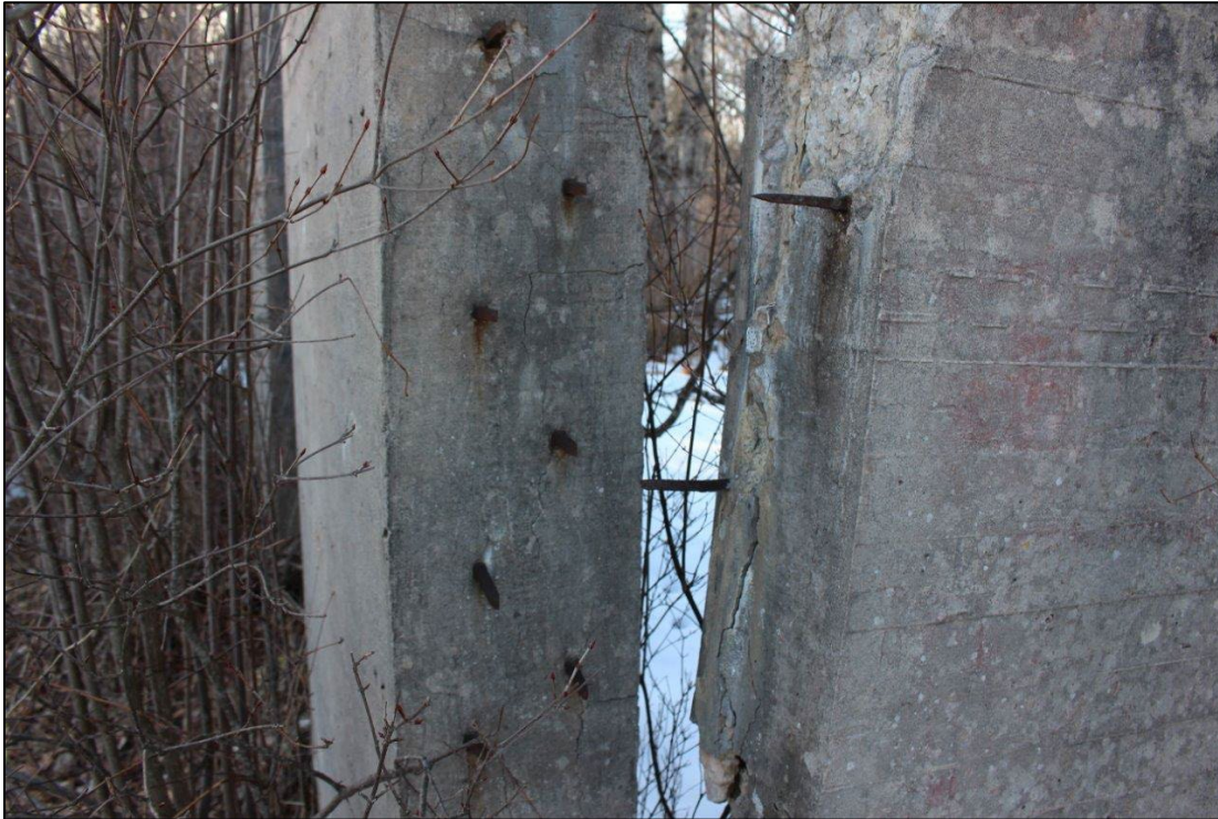
Photo 5. Building Ruins showing detail view of connection point between concrete slabs, facing northwest.
