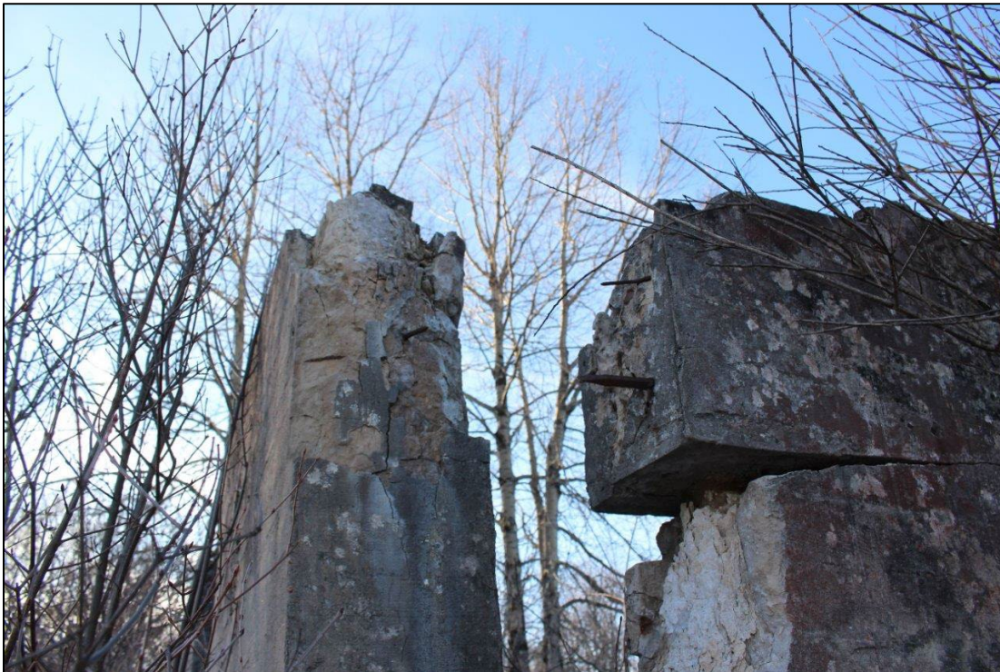
Photo 6. Building Ruins showing detail view of deteriorated concrete slabs, facing northwest.
