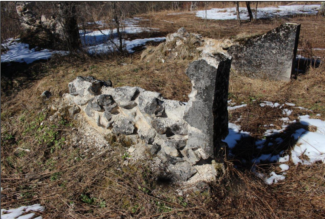
Photo 4. Detail view of gas tank foundations showing severe concrete deterioration, facing north.
