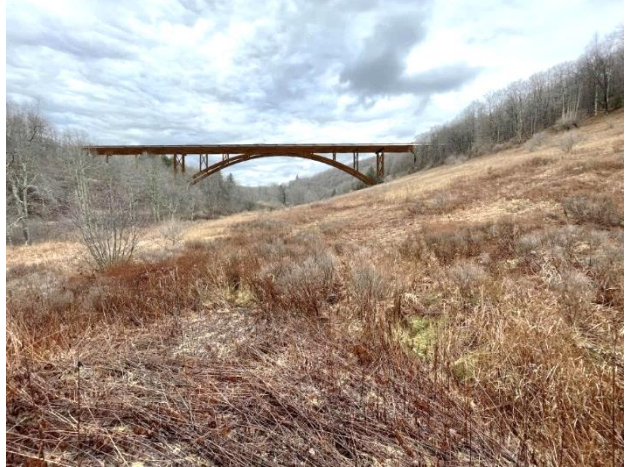
Figure 8. 2023 conceptual rendering looking toward the proposed metal arch bridge from a coke oven bank, facing north. Note the additional space along the valley floor due to the arch design reducing the incursion within the district and its viewshed.
