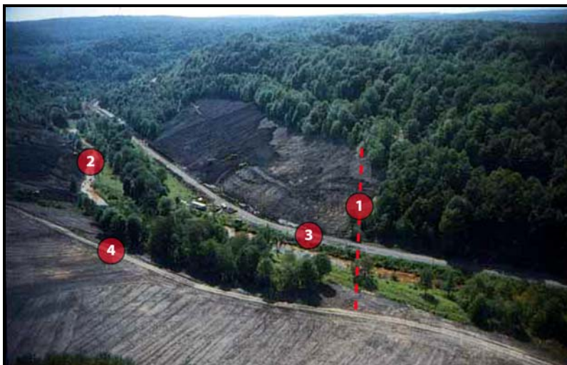
Figure 13 August 1993 view (post Douglas and Albert Highwall Reclamation Projects) of the a portion of the Blackwater Industrial Complex and approximate ROPA bridge location.. (Note the recontoured hillsides in this post-reclamation photograph. The Powerhouse Site lies in the clump of trees at the lower right side of the photograph.)
