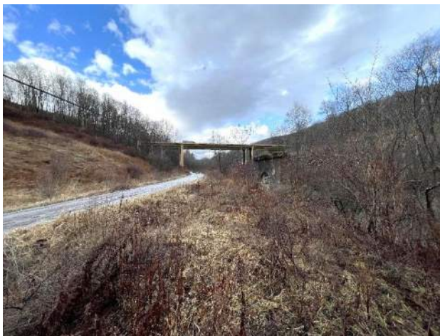
Figure 9. 2002-2007 conceptual rendering looking toward the proposed concrete box girder bridge from an area near the concrete bents of the Davis Coal and Coke Company Tipple No. 36, facing north as shown in Figure 4.
