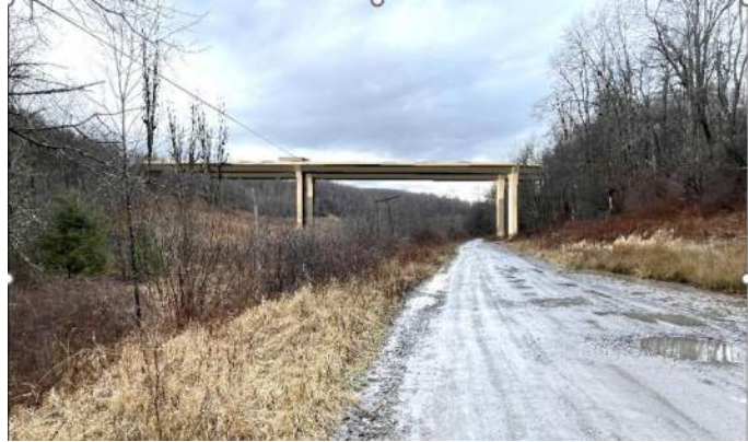
Figure 5. Schematic rendering showing the proposed 2002-2007 bridge over the Blackwater Industrial Complex looking toward the proposed concrete box girder bridge area from CR 27/3.
