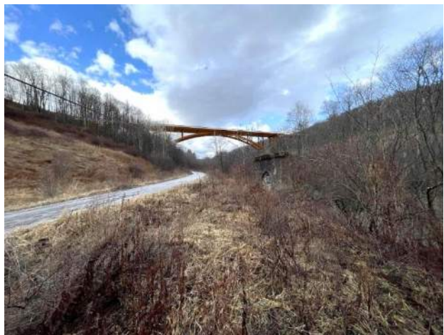
Figure 10. 2023 conceptual rendering looking toward the proposed metal arch bridge from an area near the concrete bents of the Davis Coal and Coke Company Tipple No. 36, facing north as shown in Figure 4.
