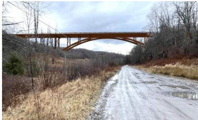
Figure 6. Schematic rendering showing the proposed 2023 bridge design over the Blackwater Industrial Complex looking toward the proposed steel arch bridge from CR 27/3.
