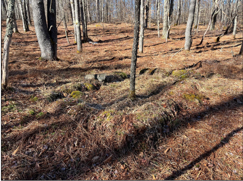
Figure 15: View of rough-cut stone foundation facing west
