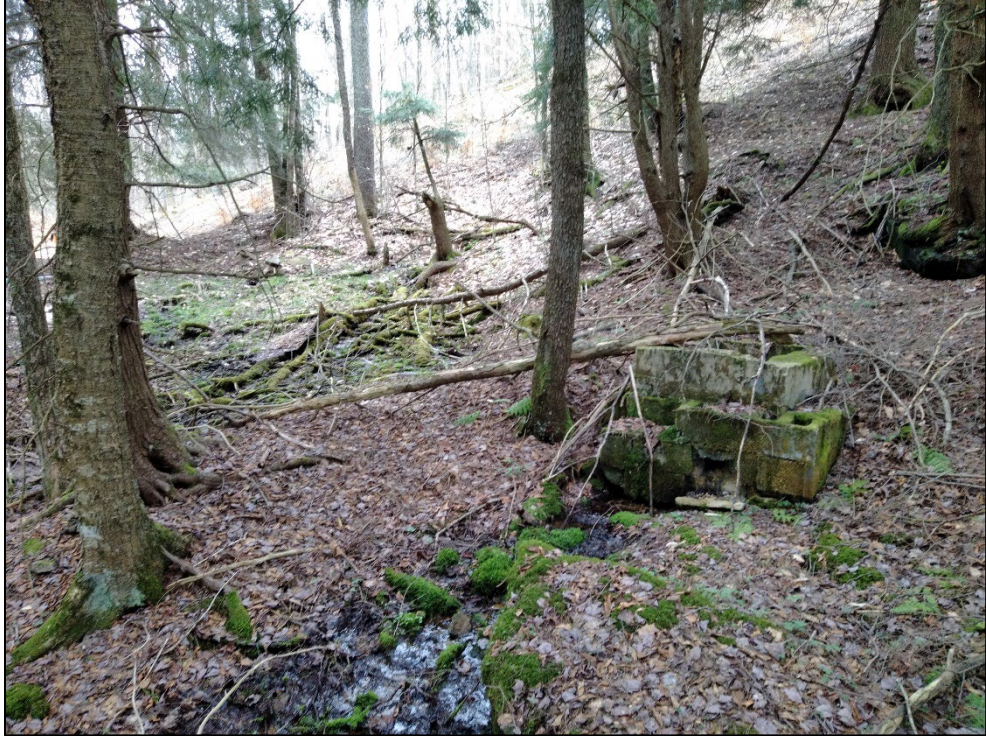
Figure 21: One of four springhouses in the vicinity of the proposed US 219 interchange at Thomas
