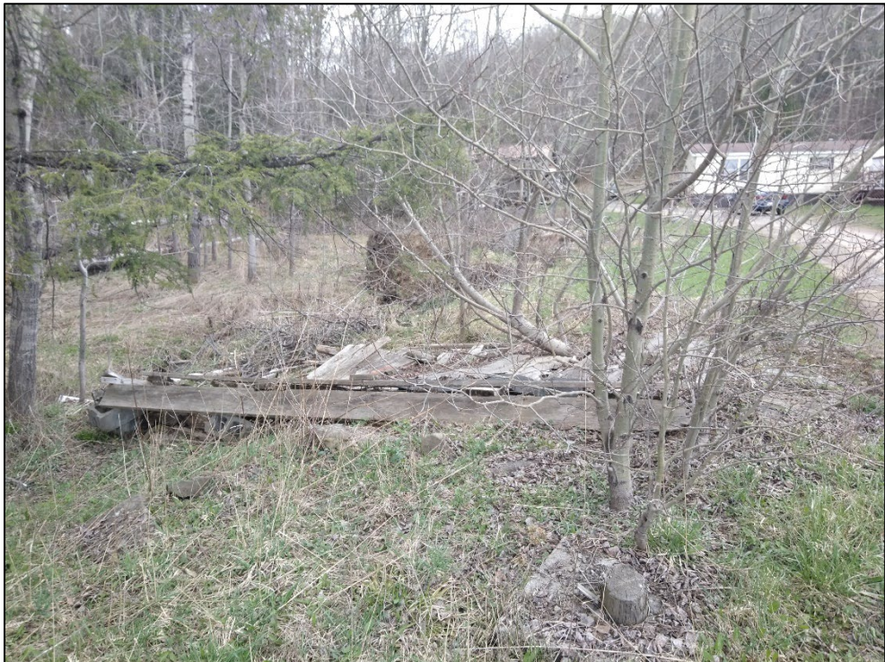
Figure 22: View facing east showing foundation and structural remains in the vicinity of the proposed US 219 interchange at Thomas
