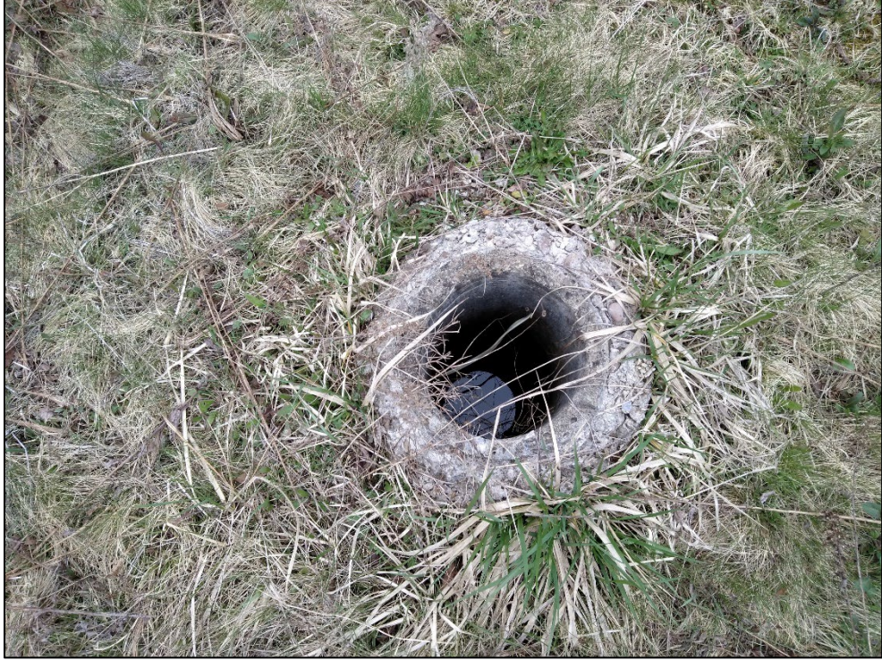
Figure 25: Plan view of orifice of concrete feature
