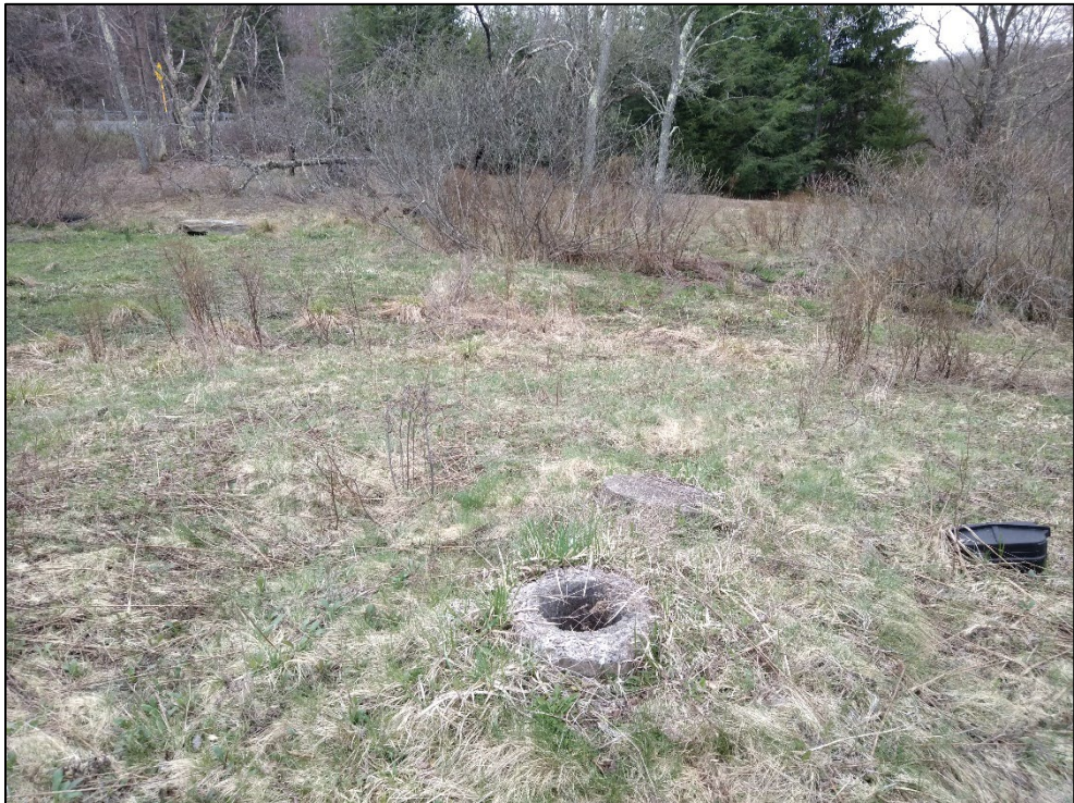
Figure 24: View of semi-subterranean concrete feature
