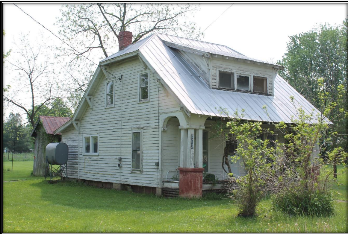
Photograph 8. HY-0299 (463 Sand Field Road, Wardensville), facing southeast.
