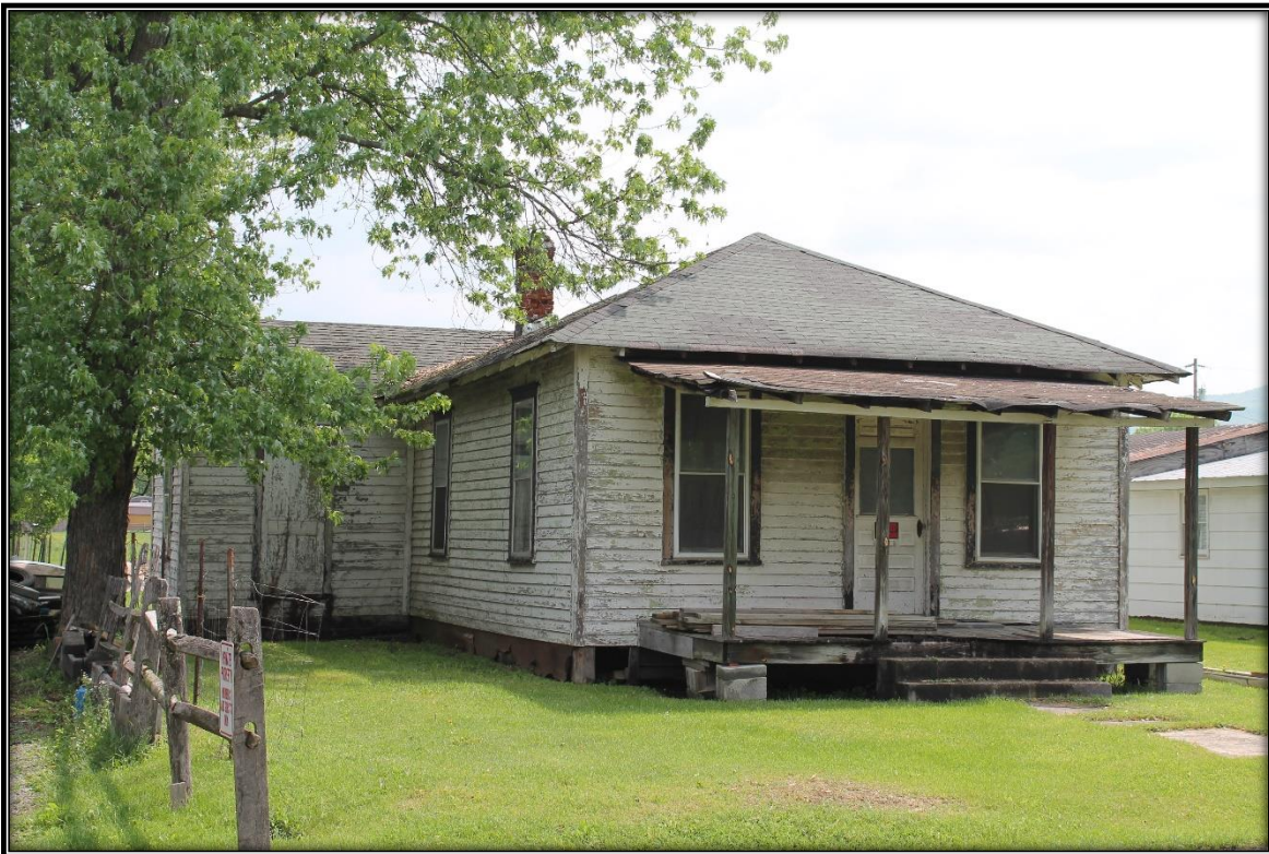
Photograph 4. HY-0871 (397 Sand Field Road, Wardensville), facing southeast.
