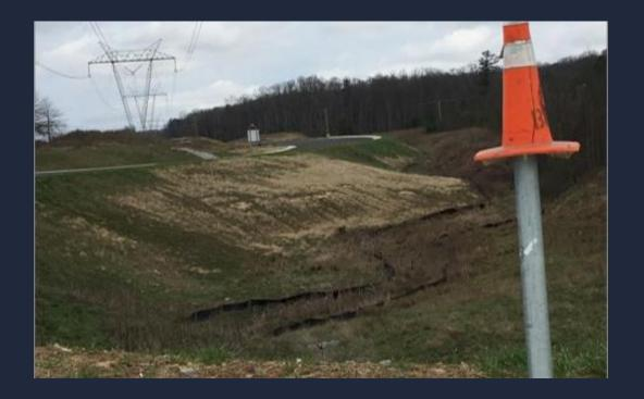
Install on the contour perpendicular to the flow of water
