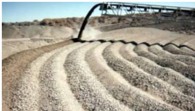
Figure 11 - Building a Stockpile using a Telescoping Conveyor
