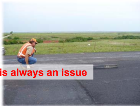
Rolling Transverse Joint
