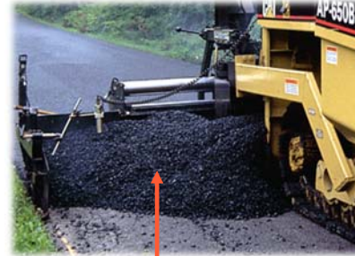
No Auger Extensions or Confinement
