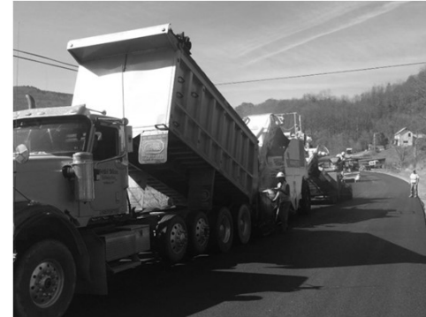
1.5" Overlay with paved shoulders
