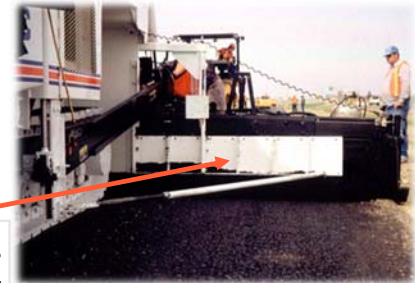
Auger Extensions & Confinement
