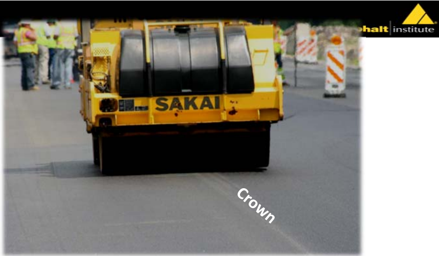
The final pass on a crowned section
