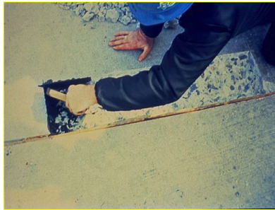
Partial-Depth Repair
