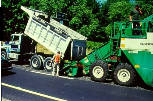
Truck dumps into MTV (rather than paver)
