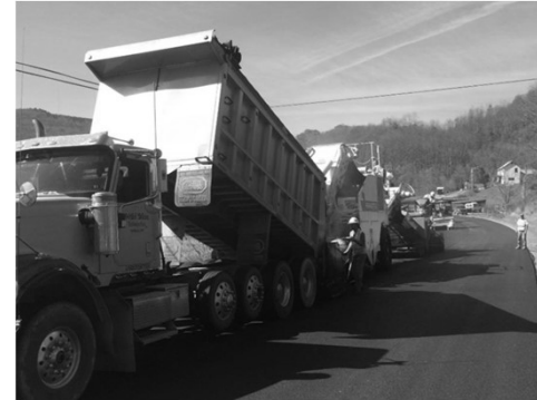
1.5" Overlay with paved shoulders
