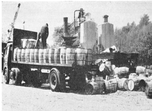
Figure 2 - Workers unloading wooden barrels of Trinidad Lake asphalt
