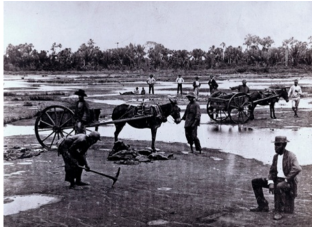
Figure 1 - Workers mining Trinidad Lake Asphalt
