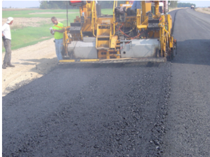
Figure 39 – Truck Segregation Effects
