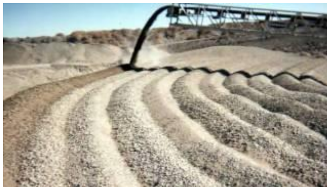
Figure 11 - Building a Stockpile using a Telescoping Conveyor
