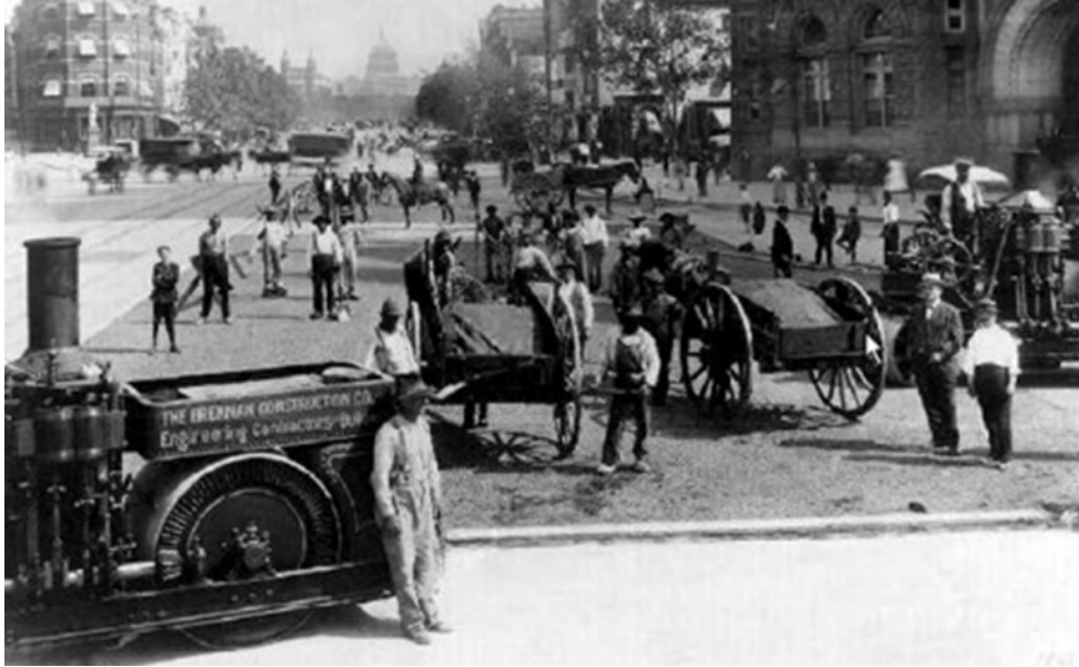
Figure 3 - Pennsylvania Ave. in Washington, DC being paved in 1876
