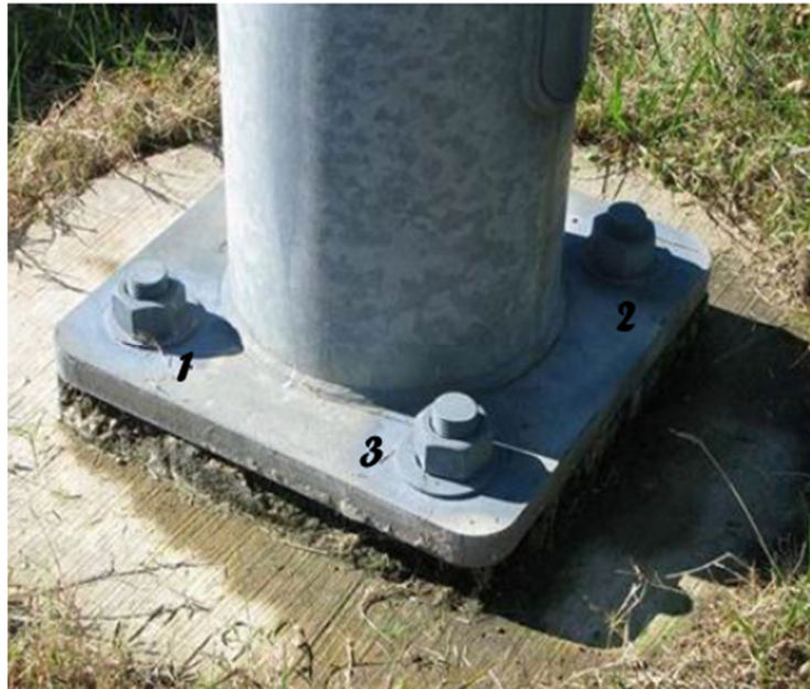
Figure 2 - Snug tightening sequence numbering on base plate.
