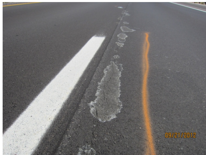
Tear in new asphalt pavement. Note water stains along cracks. Area had been marked for repair.
