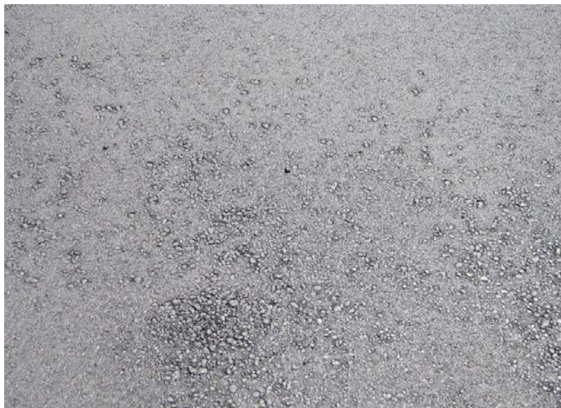
Segregation in new asphalt pavement, Superpave 9.5 mm mix.
