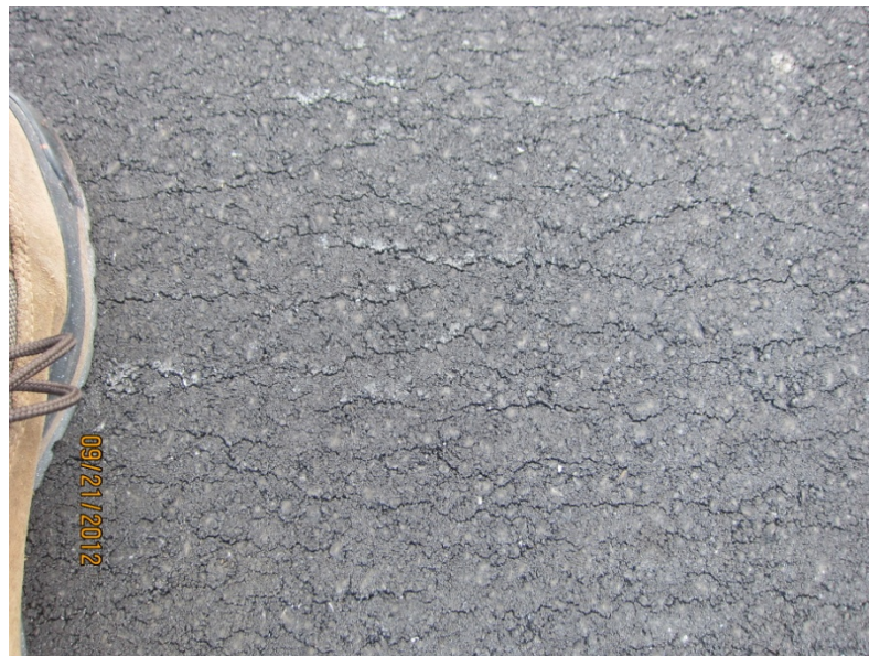
Typical observations of checking in new asphalt pavement – Superpave 9.5 mm mix.
