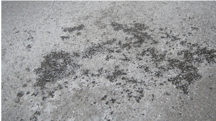
Photo shows advanced raveling and segregation of a Superpave 12.5 mm mix.
