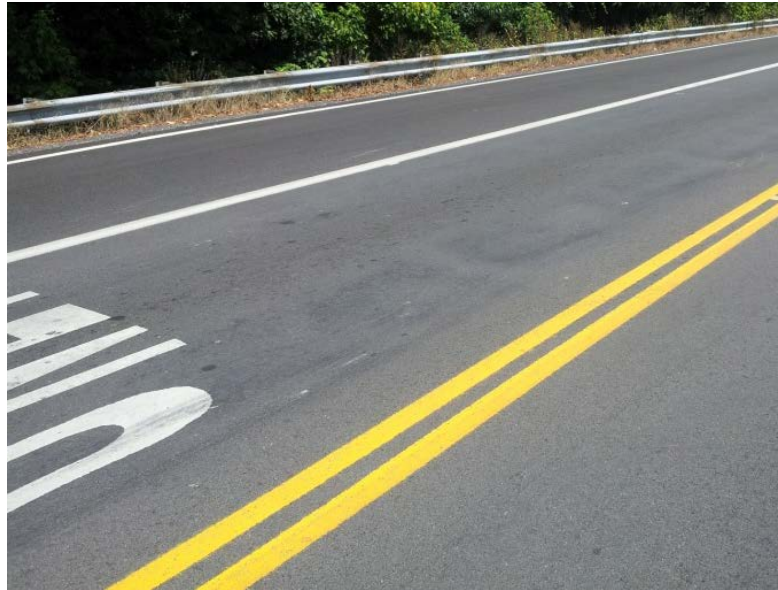
Excessive rutting and shoving in new asphalt pavement. Note the displacement of the road lettering. Also note the presence of corresponding flushing of liquid asphalt.
