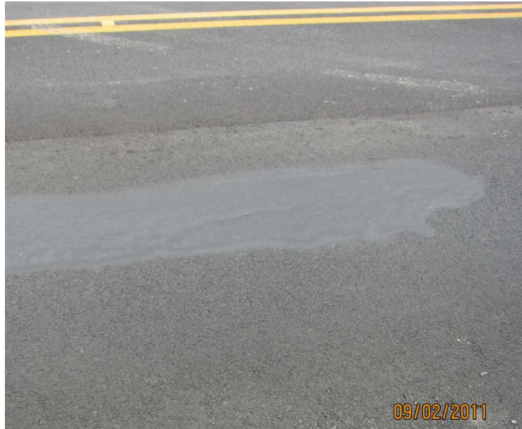
Excessive Fat Spot in new asphalt pavement.
