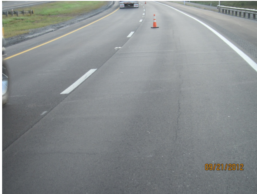
Photo showing excessive transverse bumps and associated transverse tearing as well. This photo also shows longitudinal cracking in the center of the mat.
