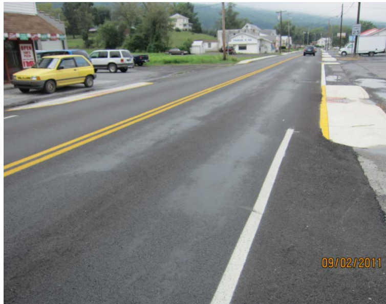
Excessive Bleeding and Flushing along wheel paths in new asphalt pavement.
