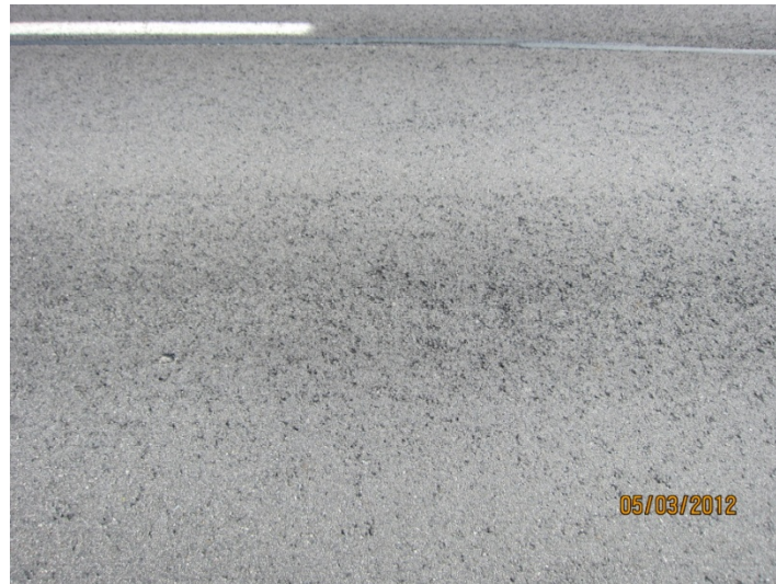
Photo shows excessive raveling of pavement within an area of segregation during first year of service – 12.5 mm Superpave mix.
