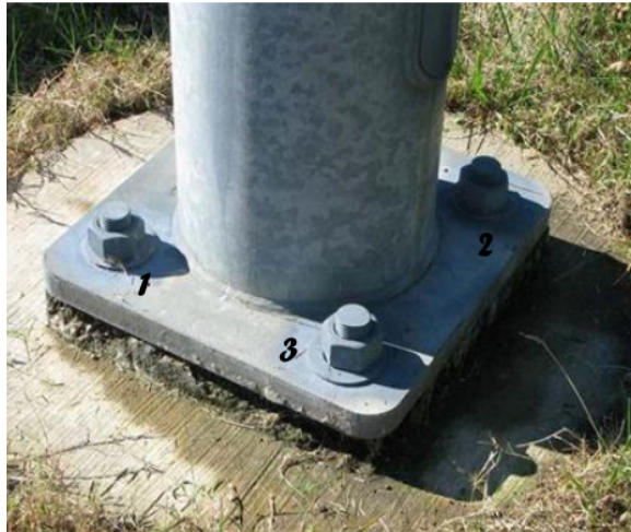
SNUG TIGHTENING SEQUENCE NUMBERING ON BASE PLATE
