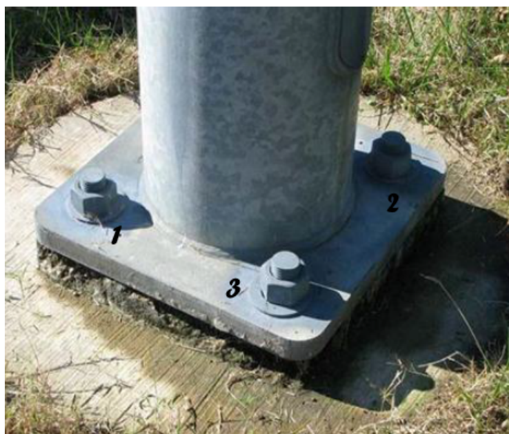
Figure 2 -Snug Tightening Sequence Numbering On Base Plate
