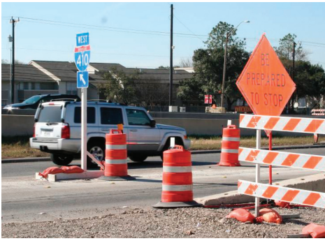
Set-up of traffic control exposes workers to public traffic
