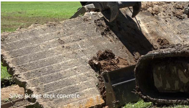
WVDOH works to retrieve Silver Bridge deck pieces
