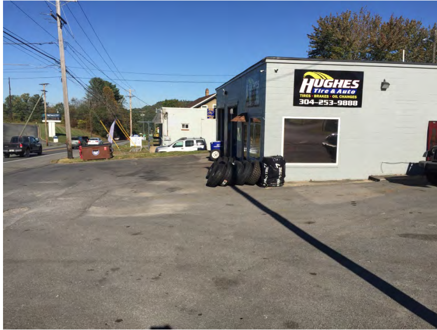
Photograph 25: View facing northwest showing the Hughes Tire and Auto and former Berton Bailes Daniels Gulf property.
