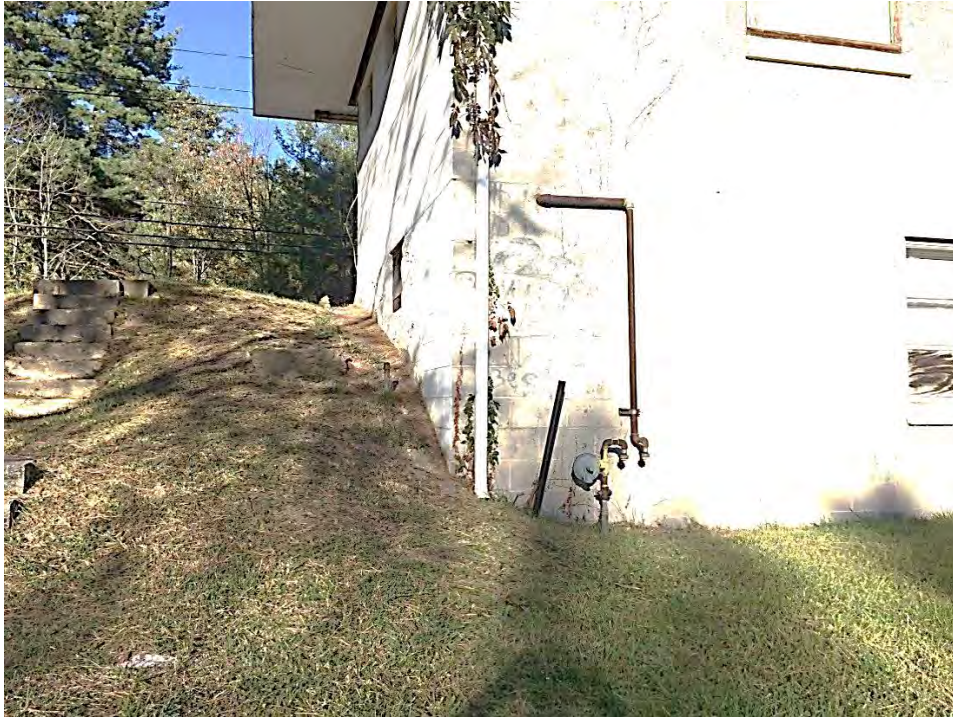
Photograph 11: View facing west showing unidentified metal pipe and cement pad located at the former Sherry's Diner property.
