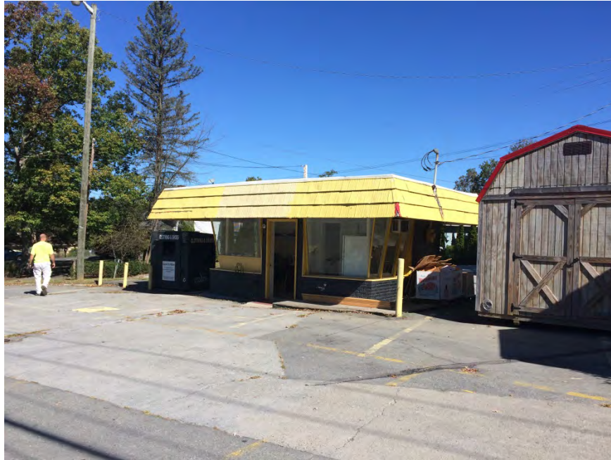
Photograph 17: View of the former Daniels Conco facility facing northwest along US-19.
