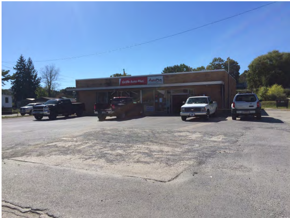
Photograph 4: View facing northwest showing Griff's Auto Parts and former Big Bear Sporting Goods (Note: rectangular shaped cement patch where the former dispenser island was located and vent lines on the north side of the building).
