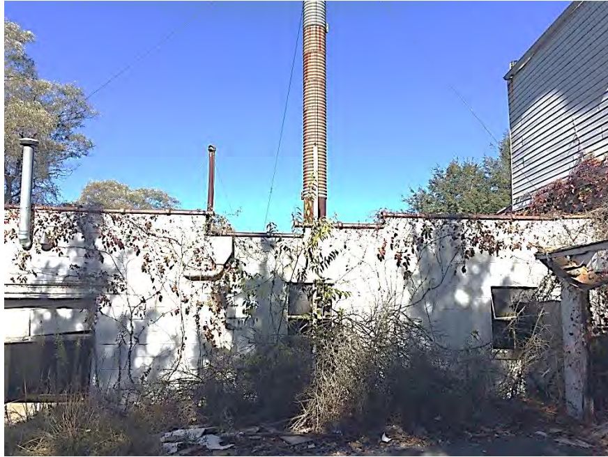
Photograph 23: View facing west of the Peerless Packaging building showing corrugated metal chimney associated with metal burner/incinerator (see below).
