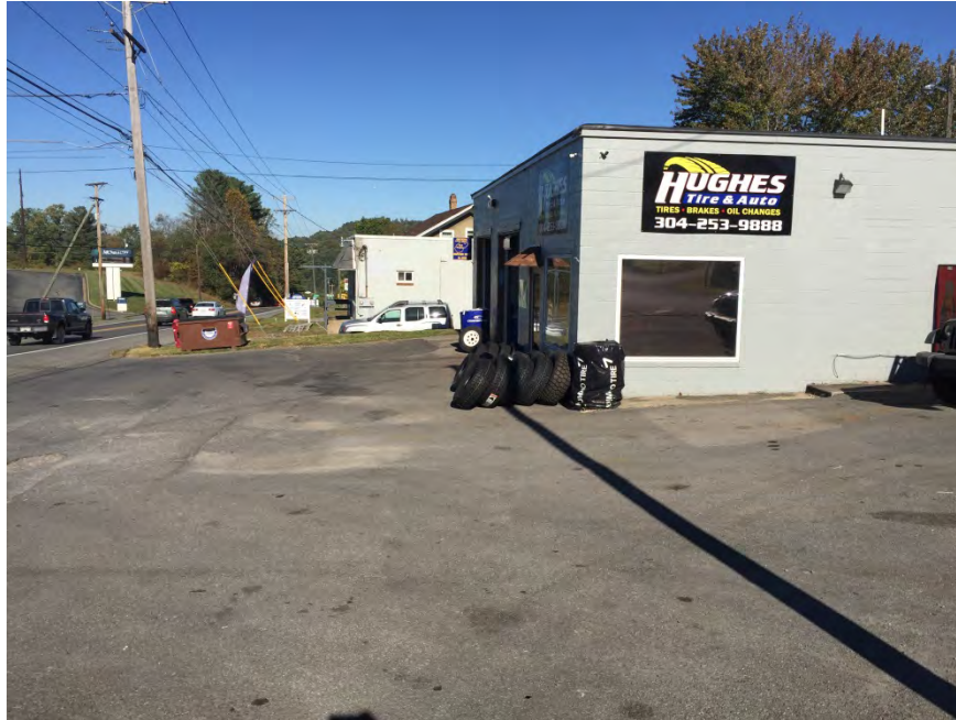
Photograph 25: View facing northwest showing the Hughes Tire and Auto and former Berton Bailes Daniels Gulf property.
