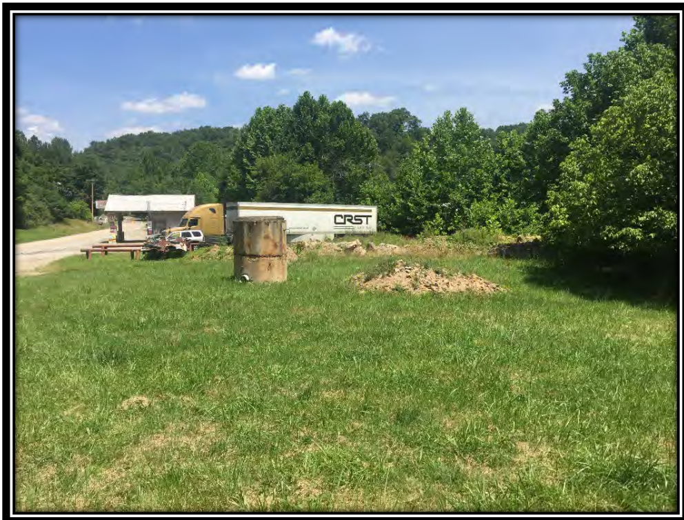
Photograph 6: View of northwest abutment area, looking from roadway. Piles of rubble and clean fill in the foreground and background.
