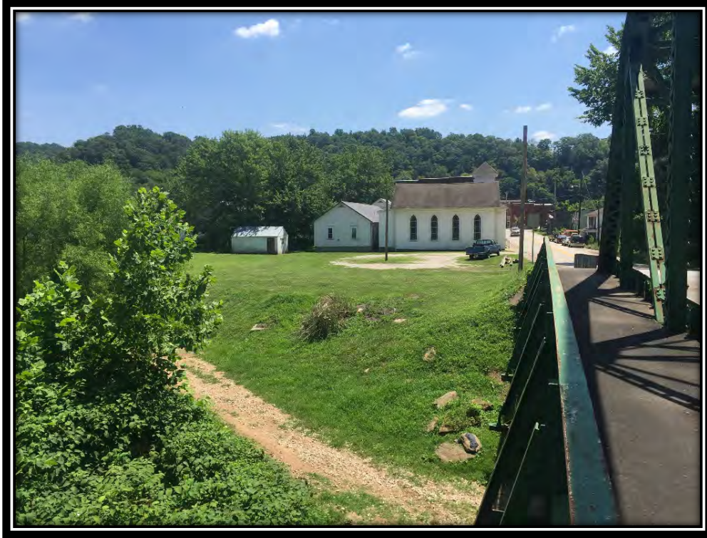
Photograph 3: View of northeast abutment from across bridge. Location of former 1900's prison; current day walking path.
