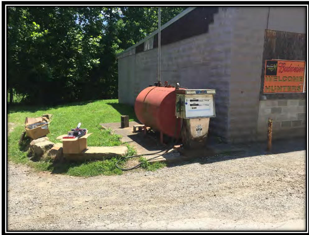
Photograph 12: AST containing dyed (off-road) diesel at the north end of The Filling Station.
