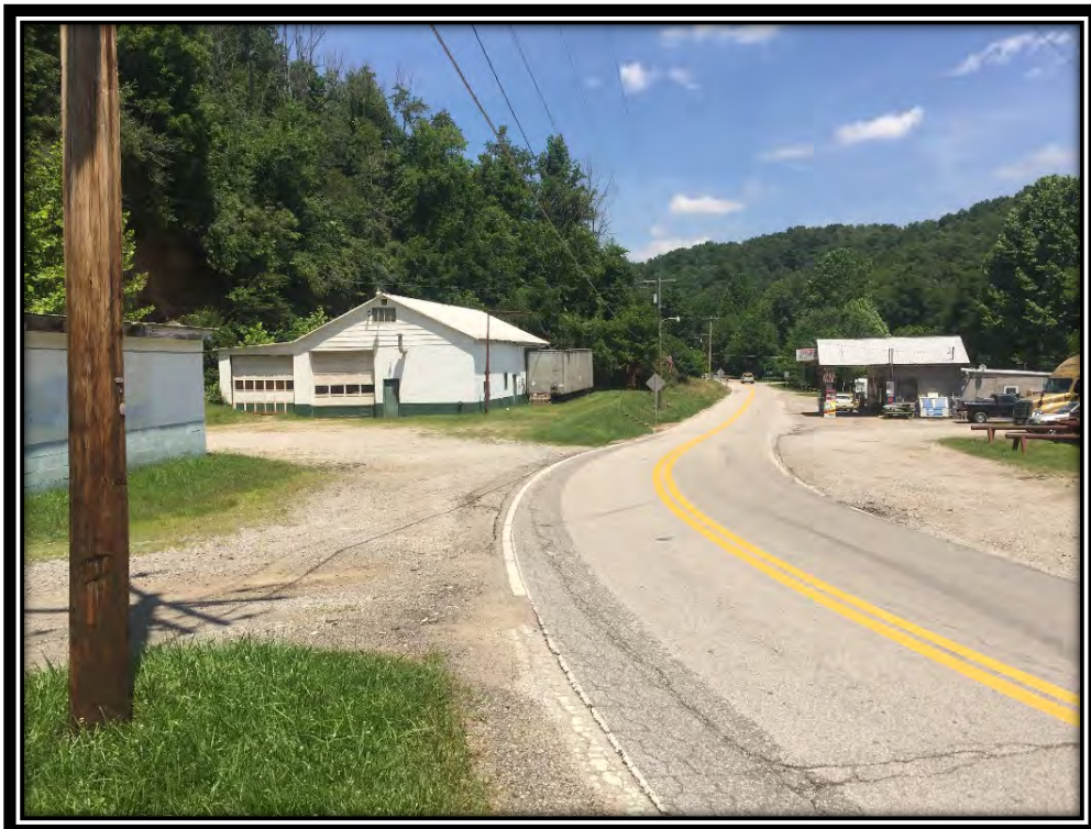
Photograph 8: View looking north on WV 31 from western end of bridge. Former car wash at left foreground, Night Owl Oil at left background, and The Filling Station at right background.
