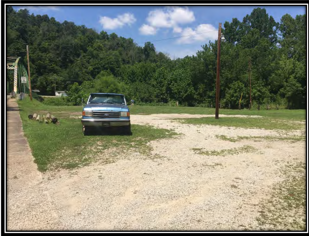
Photograph 1: View of parking lot adjacent to northeast bridge abutment (bridge on left in background).
