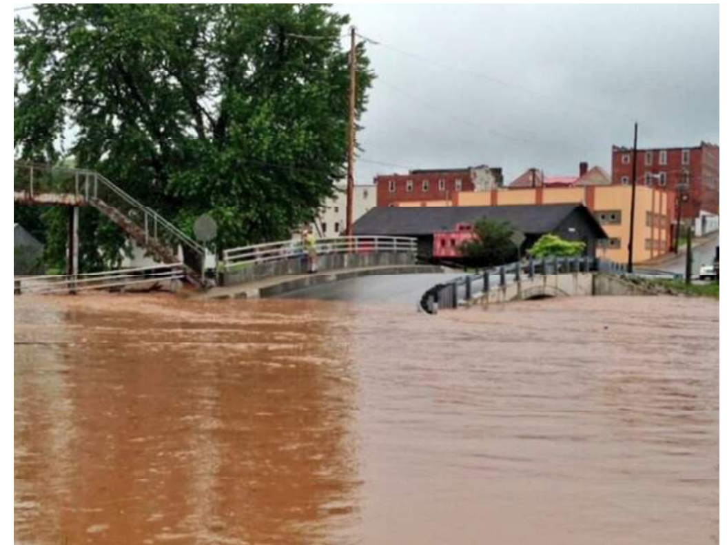
Photo 40: Flooding at North Market Street Bridge in June 2013.
