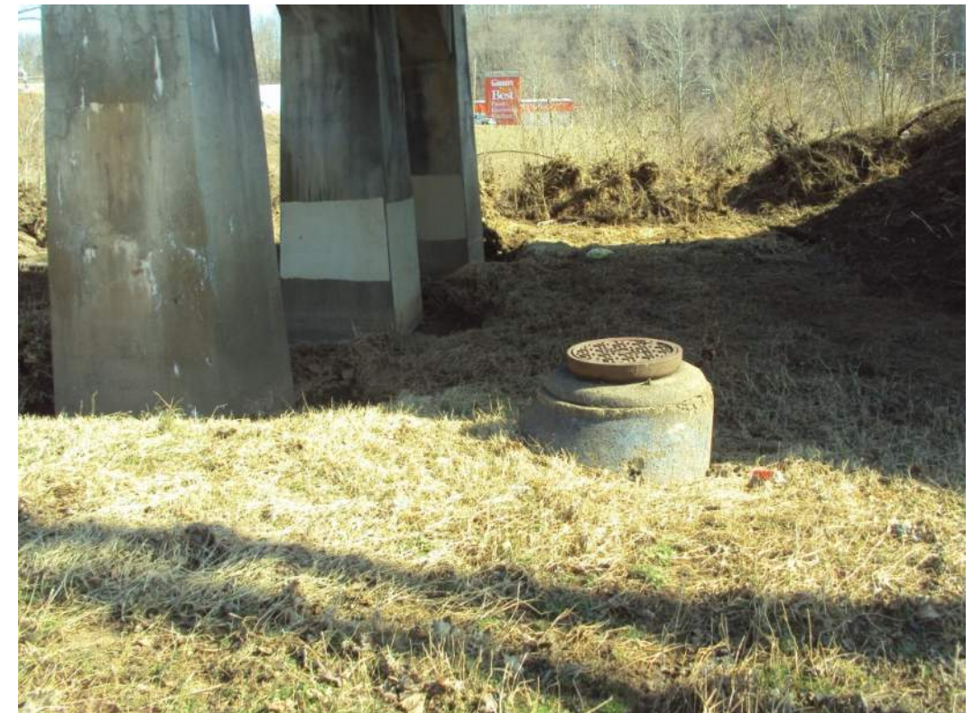
Photo 16: Sanitary manhole below Span 5 of the existing bridge.
