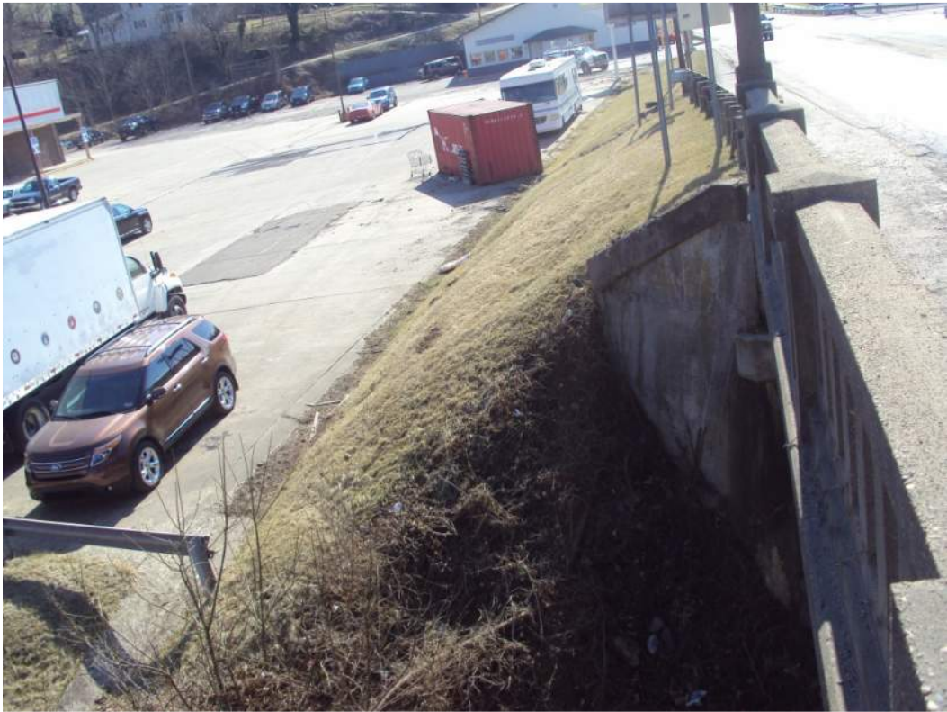
Photo 10: Save-A-Lot parking lot, adjacent to Ruby Bradley Bridge.
