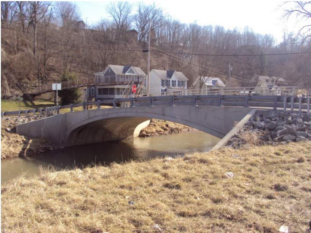
Photo 9: North Market Street Bridge.
