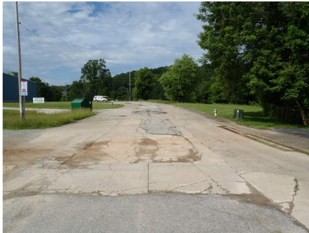
Photo 22: Looking south near match existing point on Williams Drive Extension.
