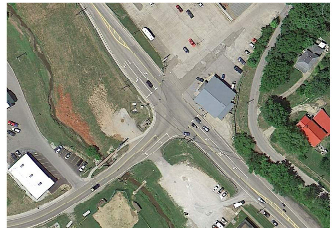
Photo 4: Turning lanes at intersection of US33 and Williams Drive.
