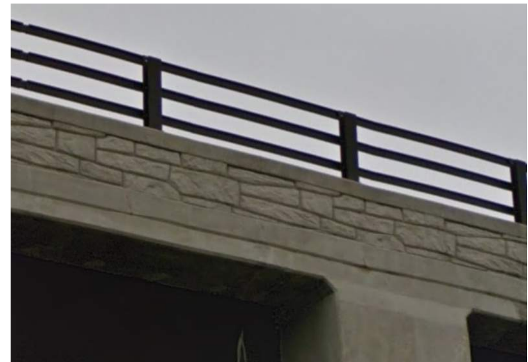
Photo 48: Close-up view of concrete stamping on Three Springs Bridge.
