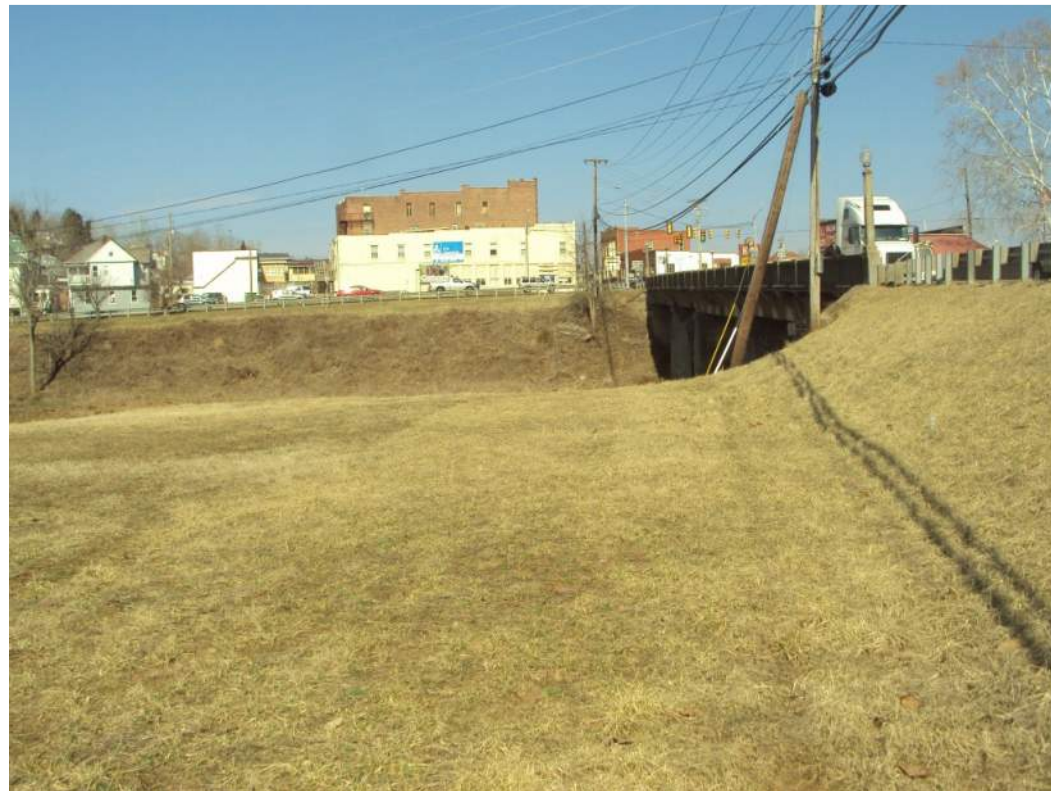
Photo 14: Upstream of existing bridge. Proposed location for Alternatives 1A, 2B and 4 temporary condition.
