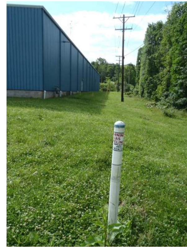
Photo 19: Gas pipeline within the proposed alignment of the Williams Extension, Alternative 3.
