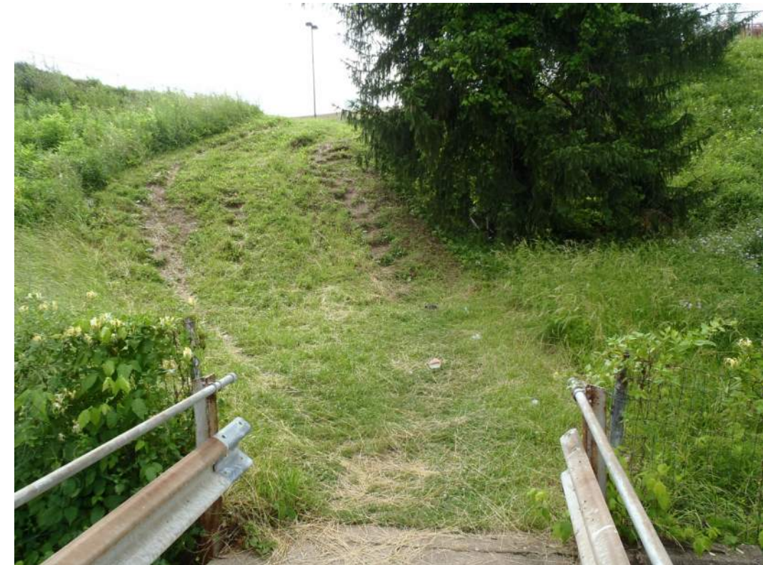
Photo 31: East approach to the existing pedestrian bridge. Note steep grade.
