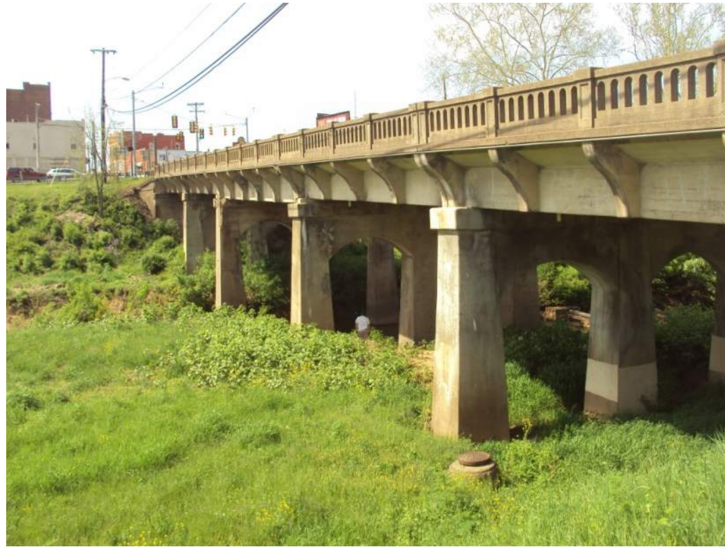
Photo 5: Existing bridge consists of CIP concrete T-beams and three-column piers.
