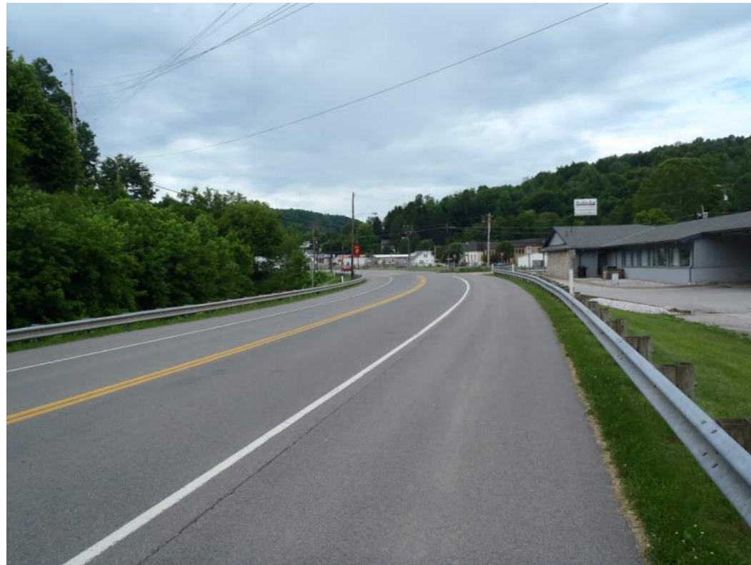
Photo 13: Typical wide shoulder along US Route 119, just north of the proposed intersection with Market Street.
