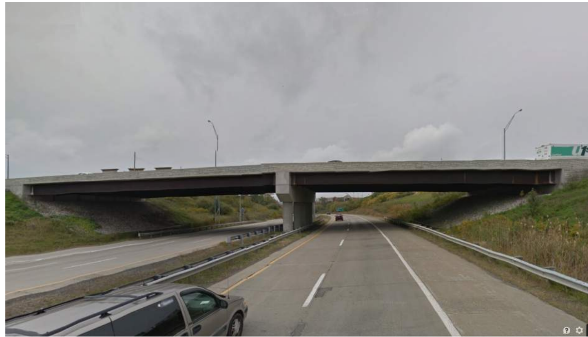
Photo 45: Elevation view of Three Springs Bridge over US 22 in Weirton, WV.
