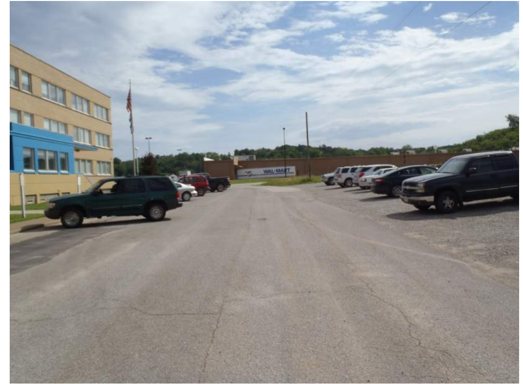
Photo 23: Looking north at Williams Drive detour route in front of Roane County Family Medical. Note head-in parking along route will need to be eliminated.
