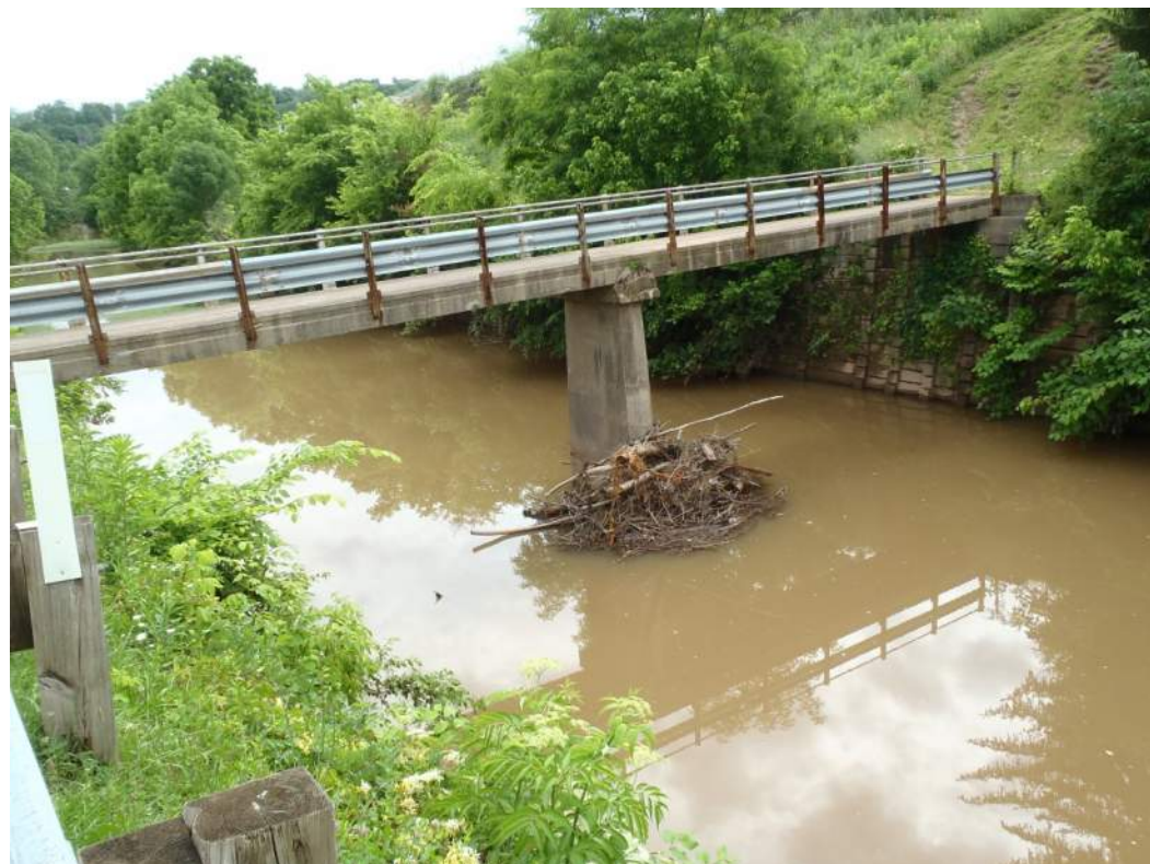
Photo 30: Pedestrian bridge adjacent to Walmart, approximately 1200' upstream from Ruby Bradley Bridge.
