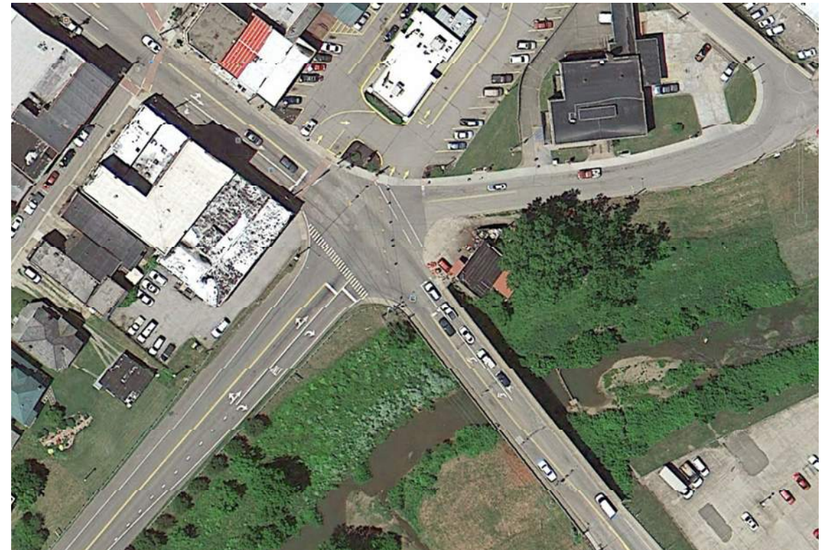
Photo 3: Aerial view of bridge and intersection of US33, US119 and North Main Street.
