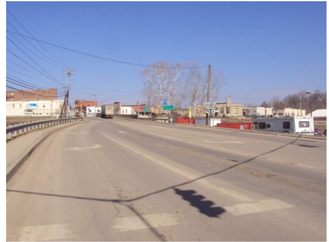
Photo 7: East approach to bridge and turning lanes at US33 intersection with Williams Drive.
