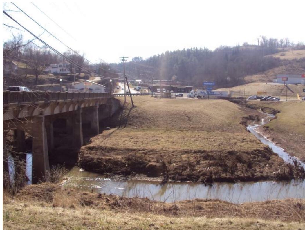
Photo 38: Upstream side of bridge. Location of required TCE for Alternatives 1A, 2B and 4, from Sisters Properties, LLC.
