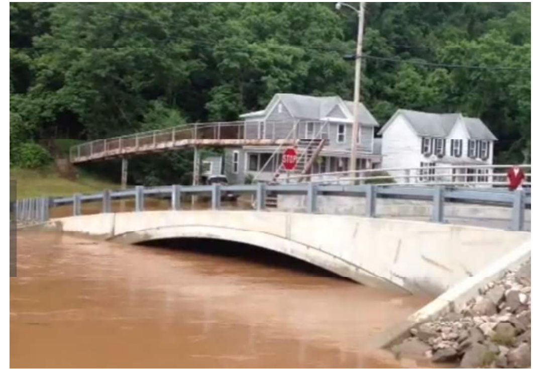
Photo 39: Flooding at North Market Street Bridge in June 2013.
