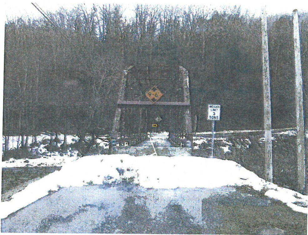
Looking West at Bridge Deck
