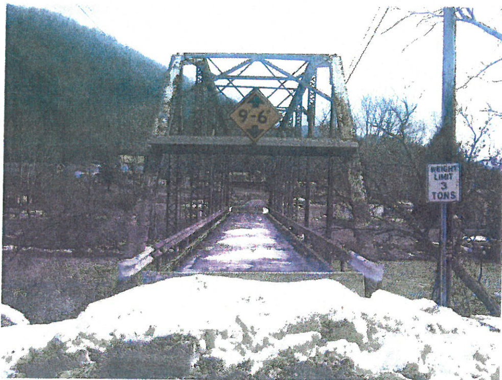
Looking East at Bridge Deck
