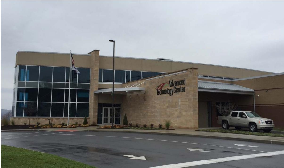
Figure 10. New (2014) Advanced Technology Center just east of the Project Area.
