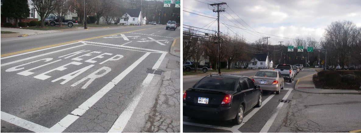
Figure 6. Two views, facing south, of Jefferson Road adjacent to the WV State Police South Charleston Detachment. Left: markings in the road to help prevent traffic from blocking emergency vehicle access to/from the facility. Right: Southbound queueing traffic from the Kanawha Turnpike intersection, blocking the entrance to the police facility.
