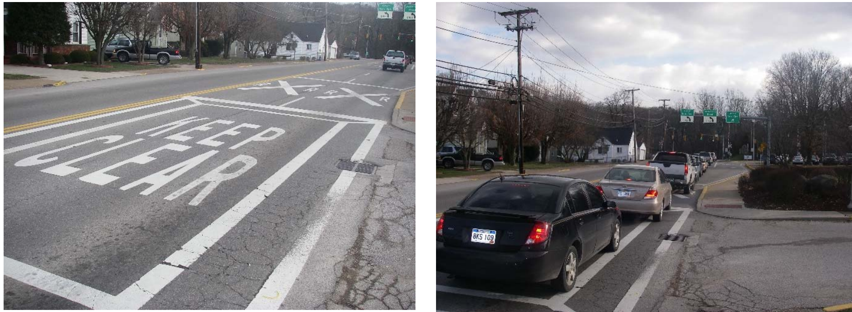
Figure 7. Two views, facing south, of Jefferson Road adjacent to the WV State Police Headquarters, South Charleston Detachment. Left: markings in the road to help prevent traffic from blocking access to the facility. Right: Southbound queueing traffic from the Kanawha Turnpike intersection, blocking the access.
