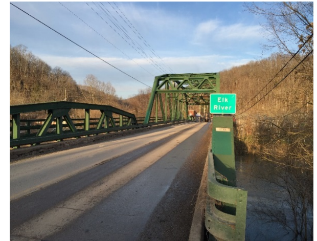
Existing Upper Gassaway Bridge facing northeast. 2/2/2016
