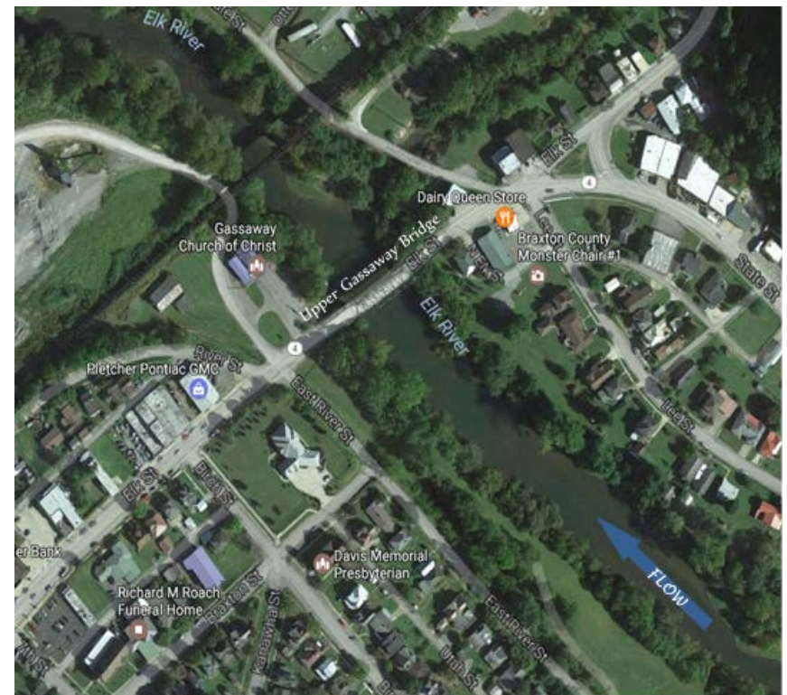
Aerial overview of Upper Gassaway Bridge crossing the Elk River, along WV-4 route
