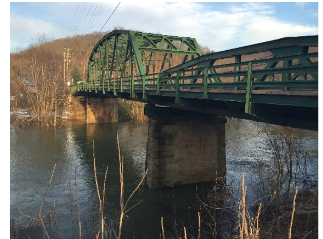
Existing Upper Gassaway Bridge facing east. 2/2/2016
