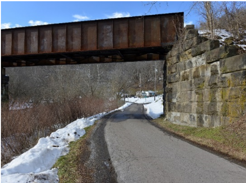
Railroad underpass on South State Street, facing northwest. 01/31/2016
