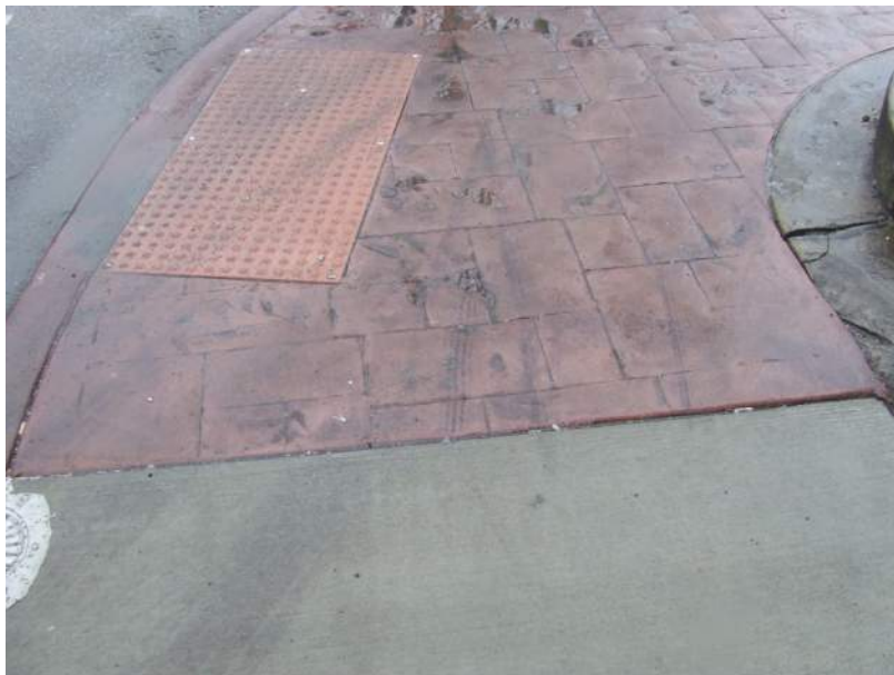
Truck tire marks on the north corner sidewalk of Madison and Chester Street
