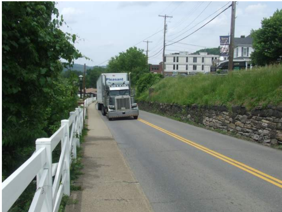
Ridge Avenue near Court Street at end of project
