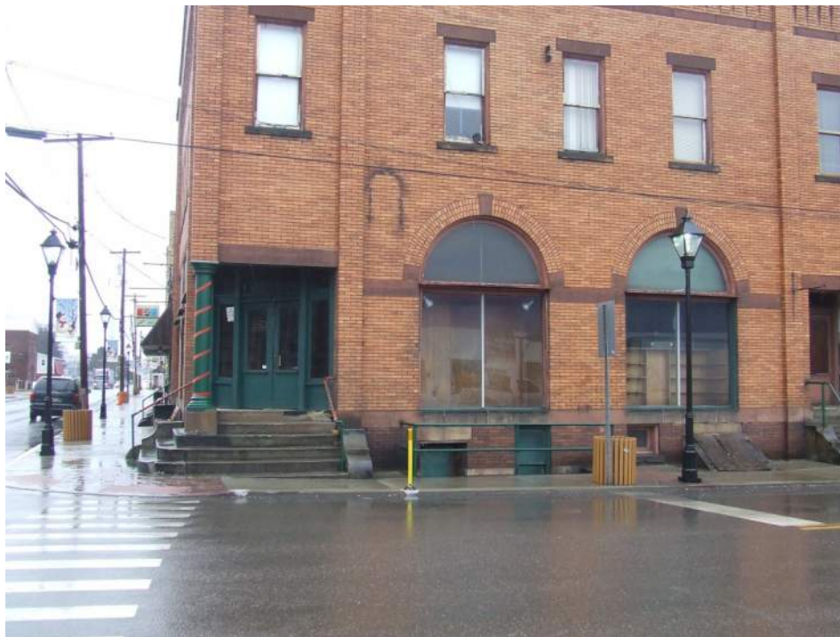
Looking north across Madison Street at historic building impacted in Alt. No. 3
